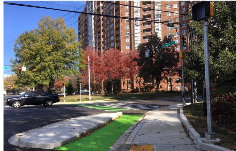
Executive Blvd Protected Bike Lanes (under construction)
