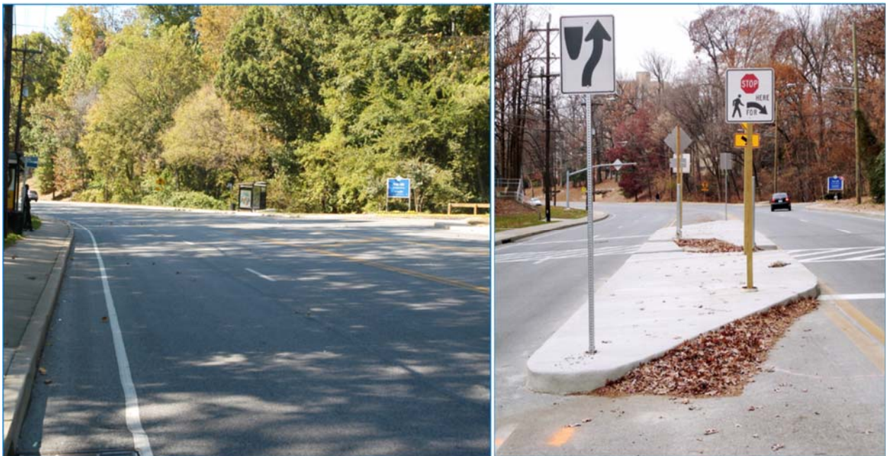
Before and After Photos of Piney Branch Road
