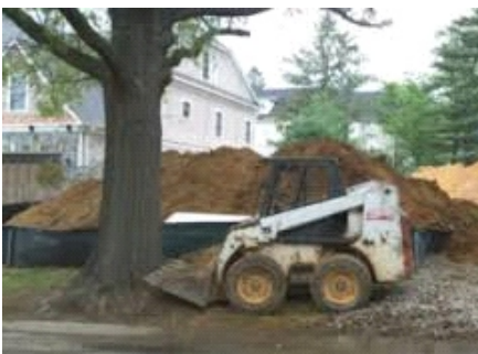
Stockpiling and parking equipment on top of roots in CRZ can cause serious harm to trunks and roots
