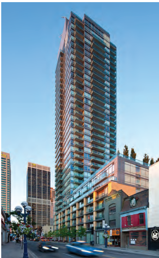
Highrise building with a base designed to relate to street and human scale Source: Architects Alliance
