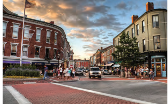
Enhanced Intersection with special paving
