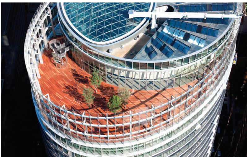
Solar power on the building roof Source: ARUP
