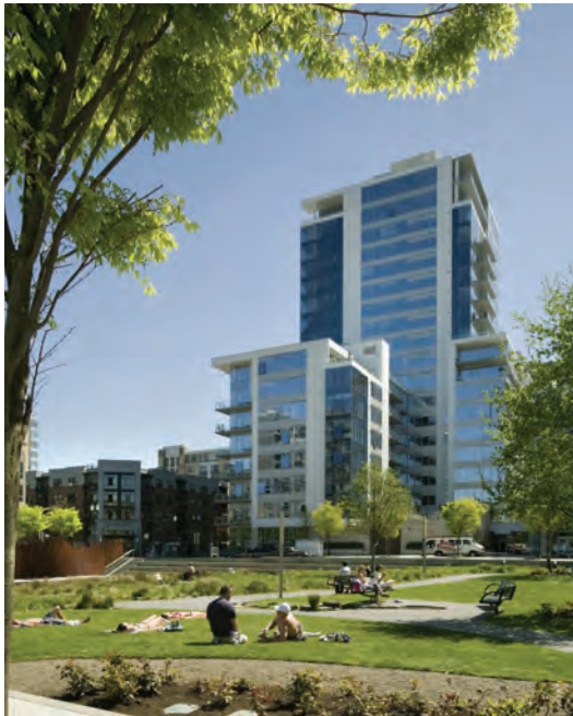
Building steps back on upper floors to protect sunlight and sky view in a public park Source: oregonlive.com
