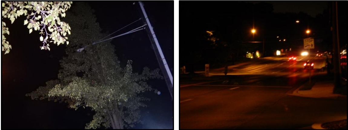
Left: Light not functioning. Right: Lighting insufficient at midblock crosswalk.
