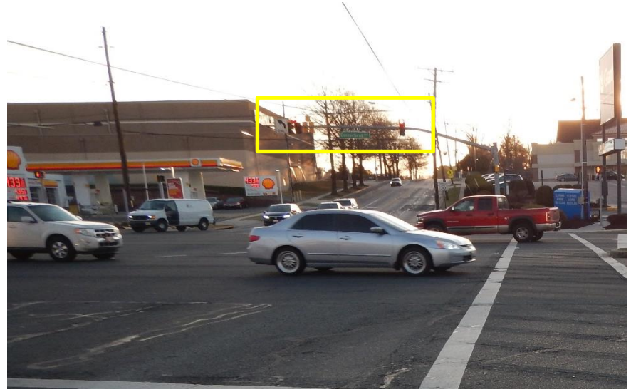
No warning signs for pedestrian and left turning vehicle conflicts (Issue 5.03)
