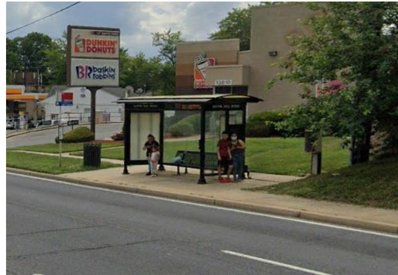
Bus shelter creates 90 degree turn in sidewalk (Issue 5.06)
