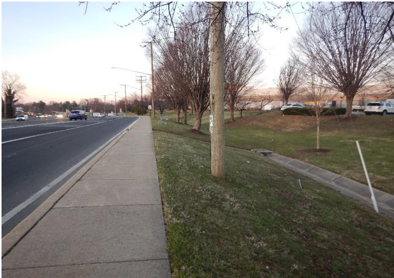
No sidewalk buffer on the west side of Connecticut Avenue (Issue 1.03)
