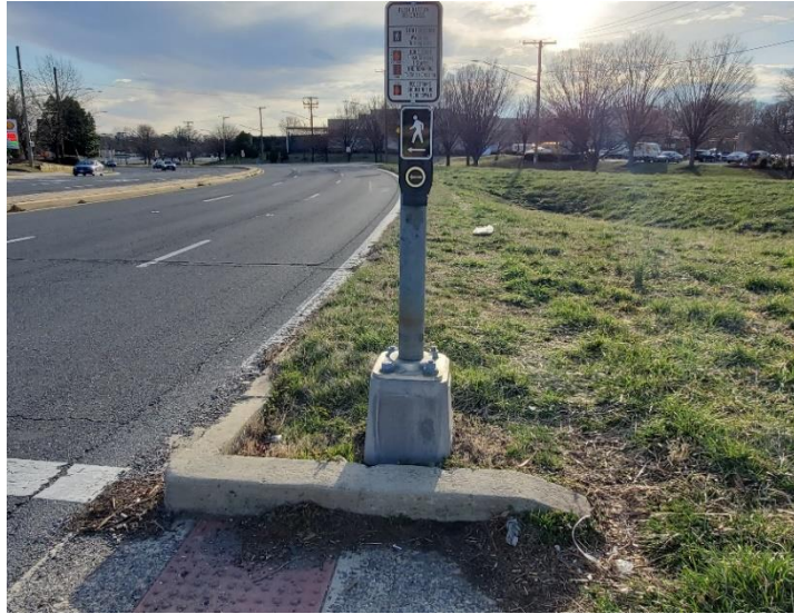
High Mounting Height for Pedestrian Push Button in Southwest Corner (Issue 2.14)
