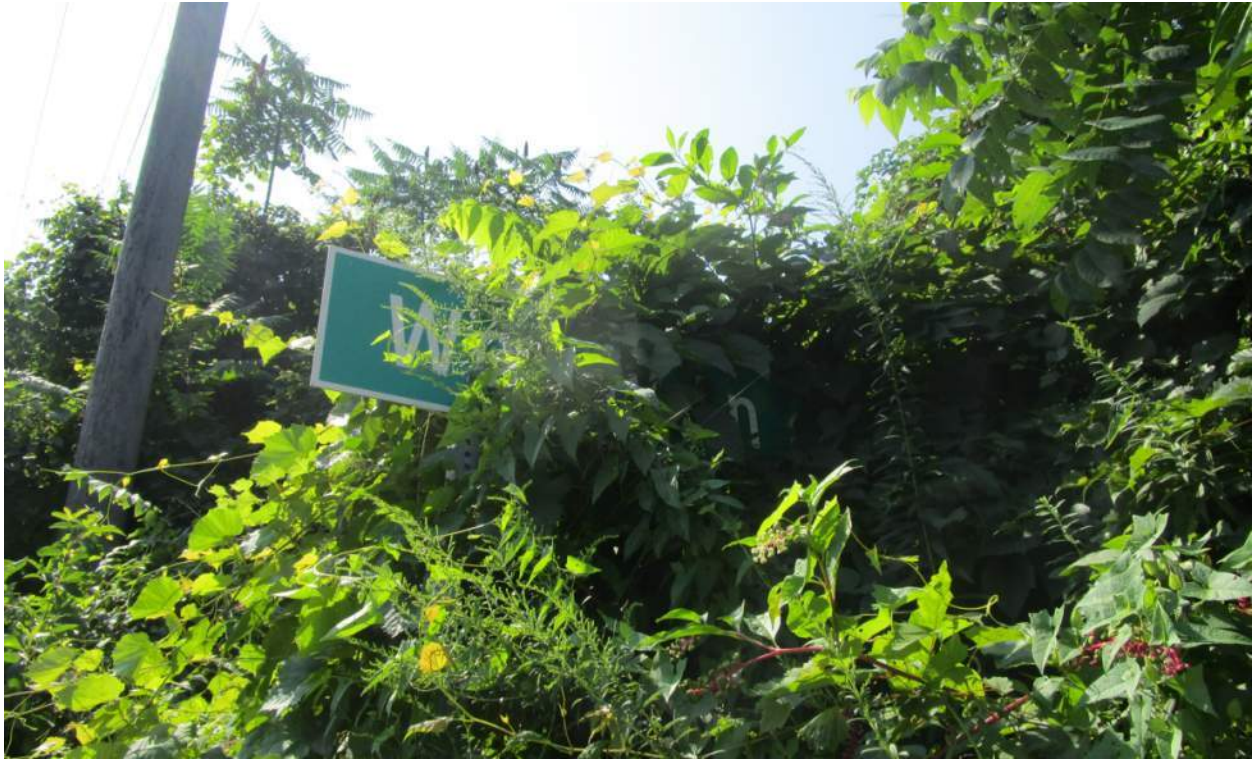
Photo 9.03. Vegetation obstructing sign visibility – SB MD 97.
