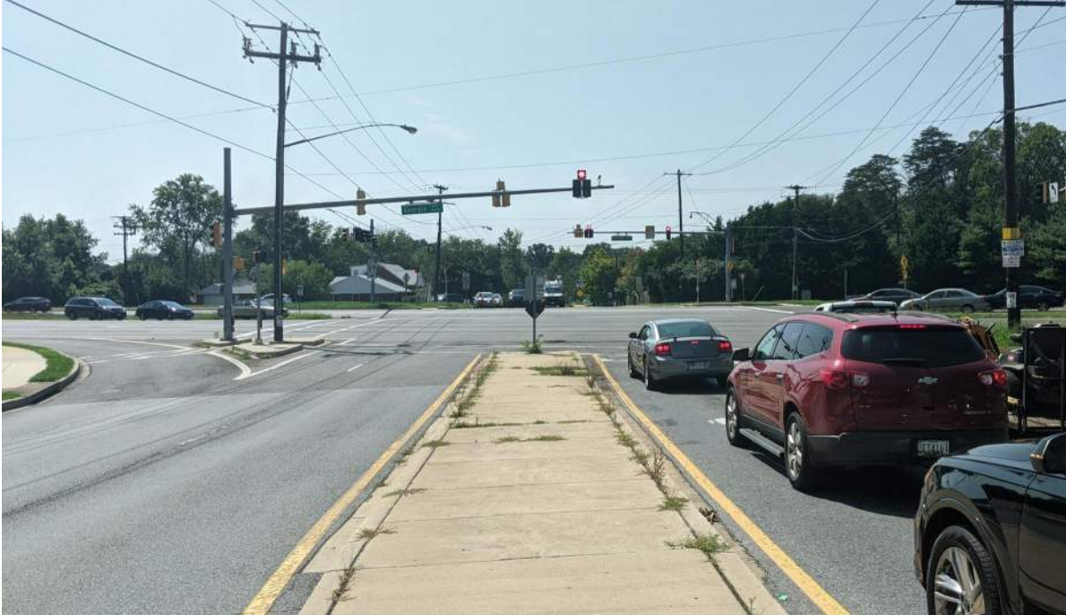
Photo 1.09. Traffic signal display – WB Bel Pre Road approach.
