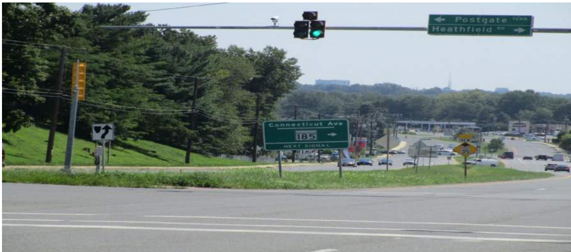
Photo 3.07. Signal heads without reflective backplates.
