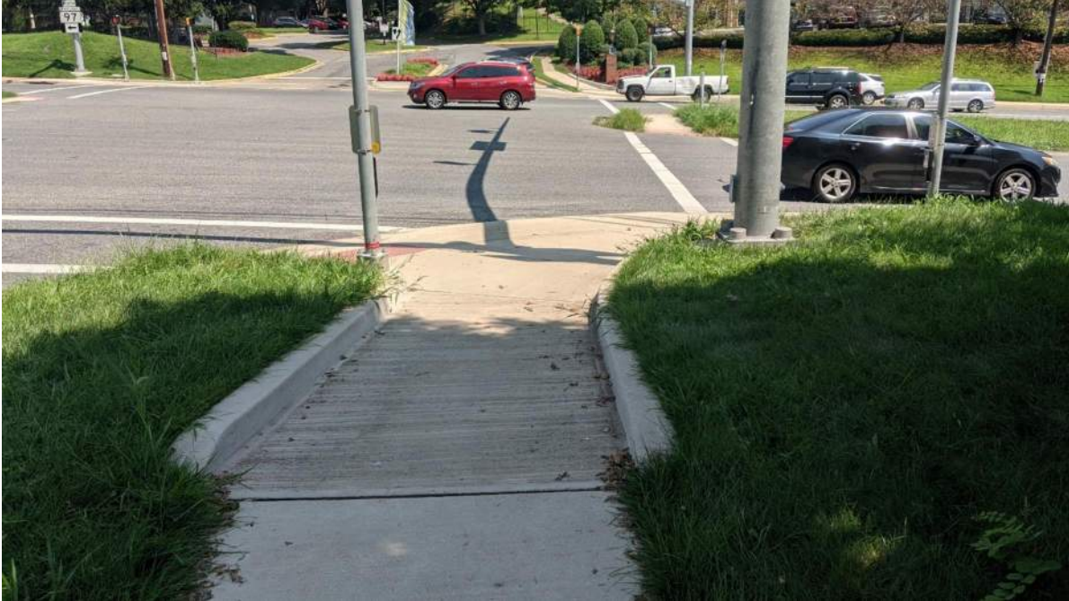
Photo 3.03. Grass sprawling into sidewalk and median at Heathfield Road.
