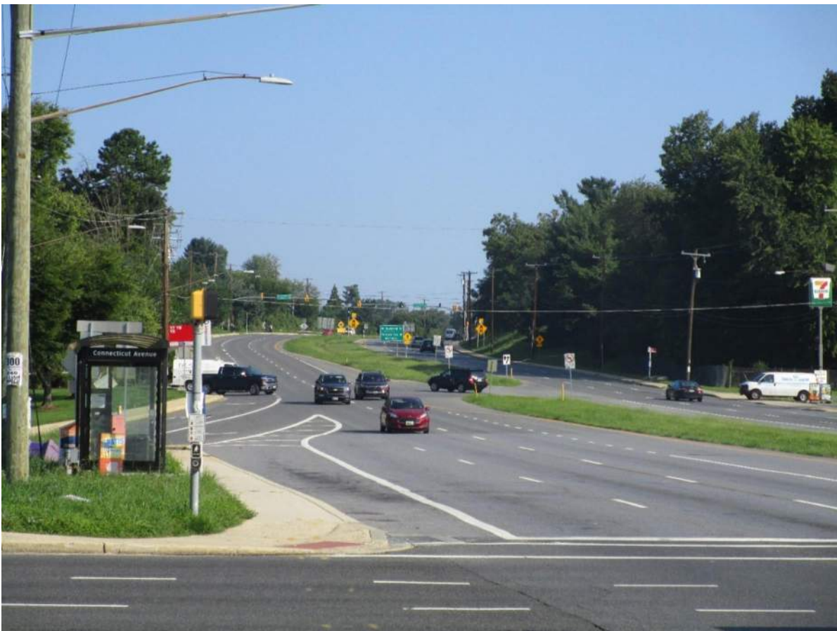
Photo 6.17. Lane configuration – SB MD 97 at MD 185.
