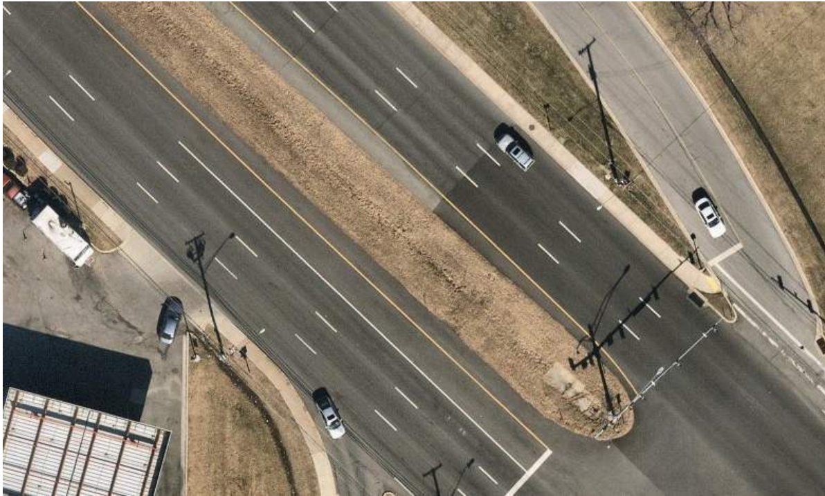
Photo 8.16. SB MD 97 left turn lane at Aspen Hill Road.
