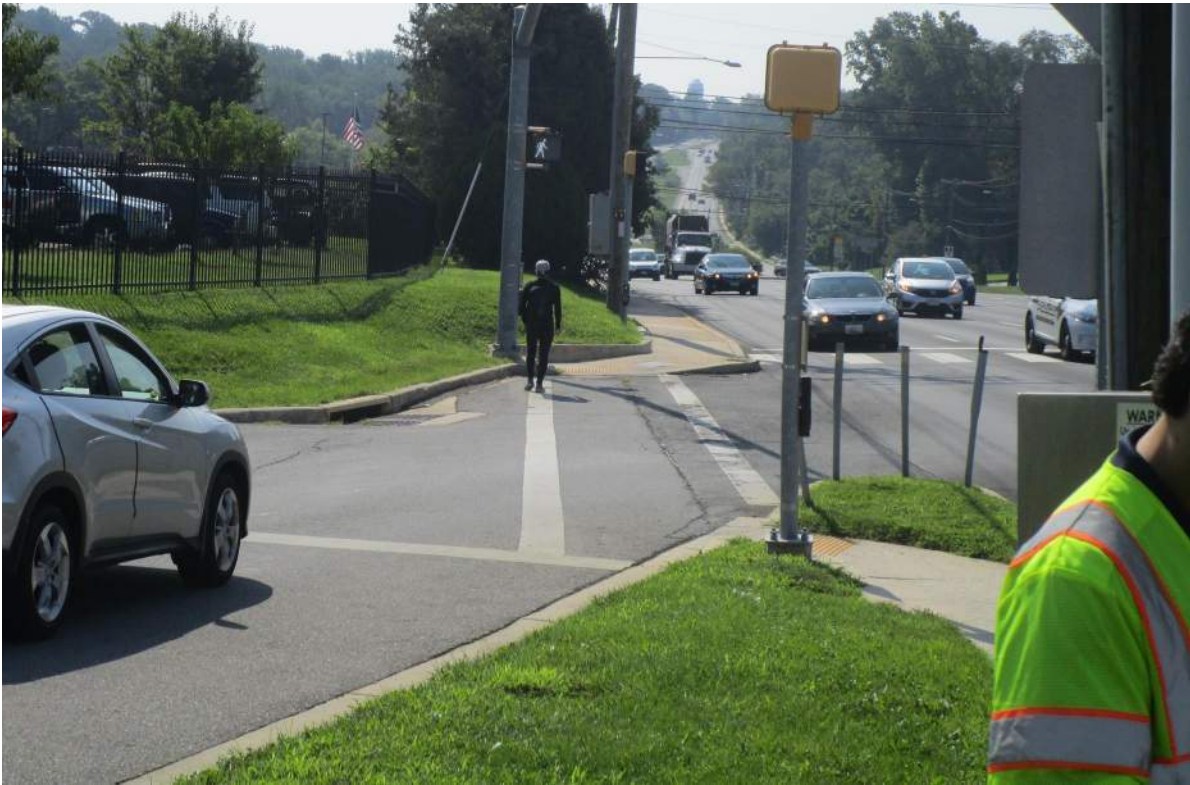
Photo 8.01. East leg crossing – Gate of Heaven Cemetery driveway.
