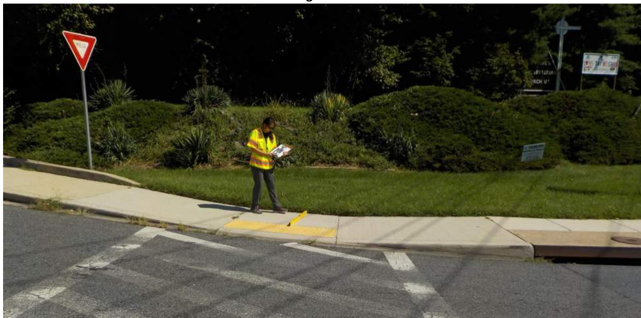
Photo 1.12. Parallel ramp in NE corner of Bel Pre Road.
