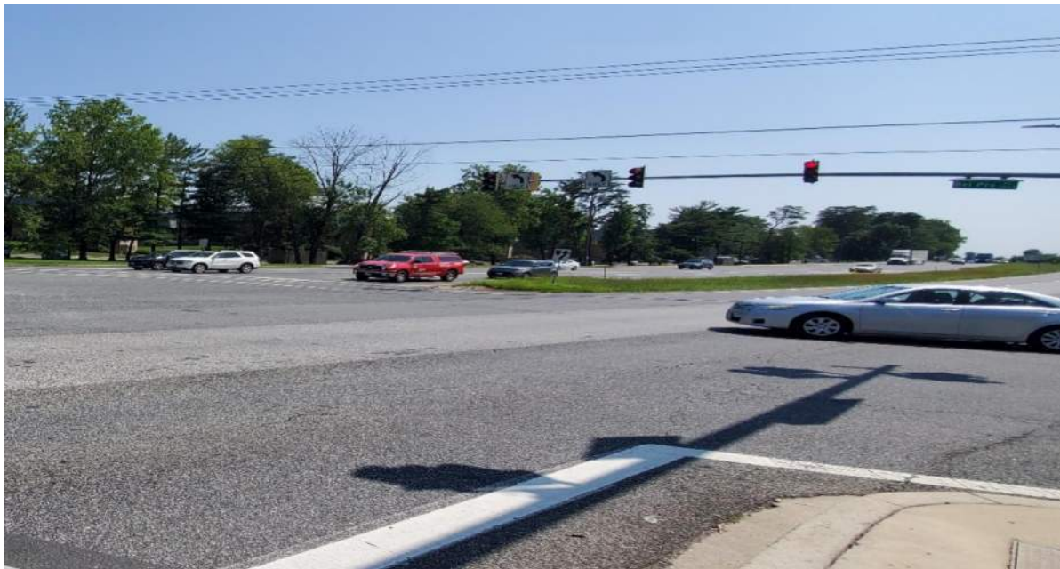
Photo 1.04. No extension lines for dual left turns – Bel Pre Rd intersection.
