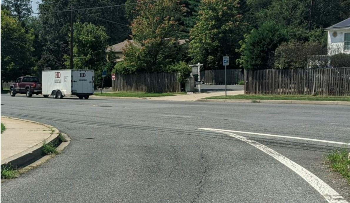
Photo 1.18. Pavement markings along west leg of Bel Pre Road.
