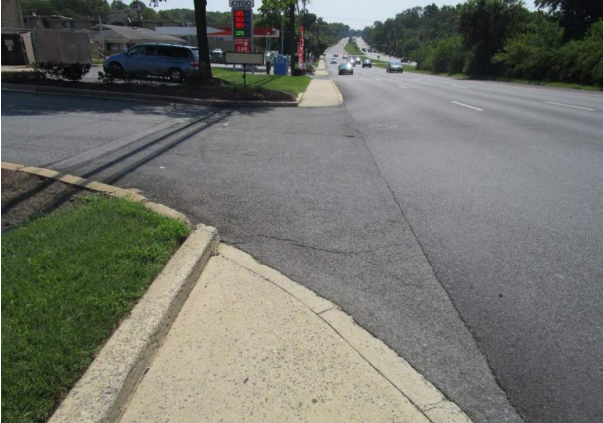
Photo 10.03. Unmarked driveway crossings along NB MD 97 for Aspen Manor / Lotte Plaza access.
