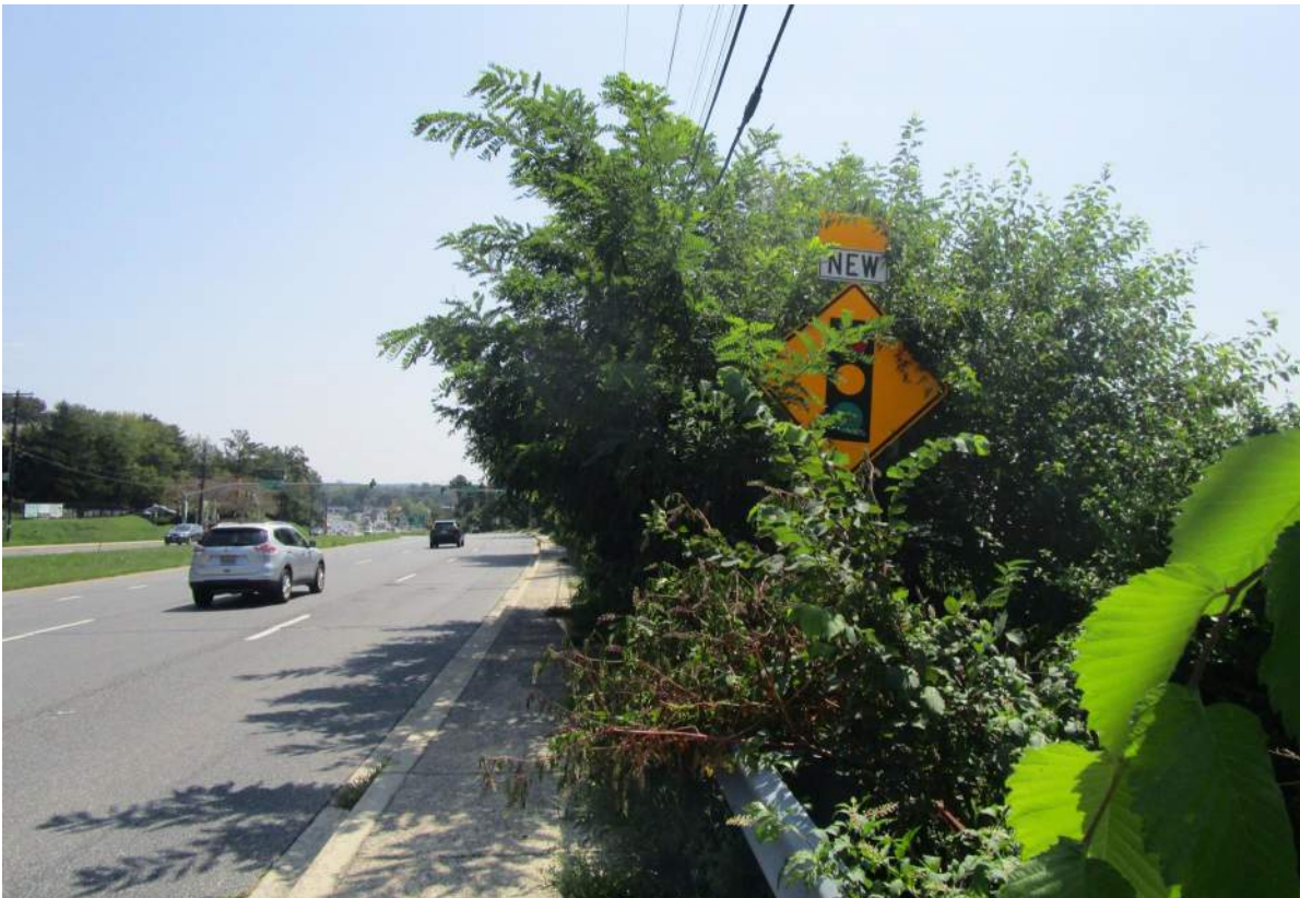
Photo 2.01. Foliage blocking signs along SB MD 97 sidewalk, south of Bel Pre Road.
