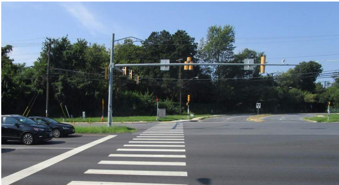
Photo 8.03. Malfunctioning CPS display – SW corner at Aspen Hill Road.
