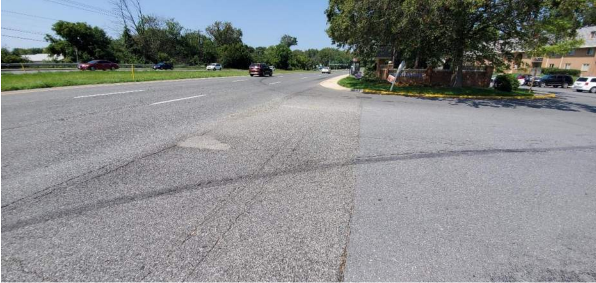
Photo 2.02. Crystal Springs Apartments driveway crossing.
