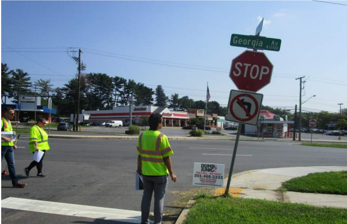
Photo 10.08. Left turn restriction supplementing stop line for Wendy Lane approach.
