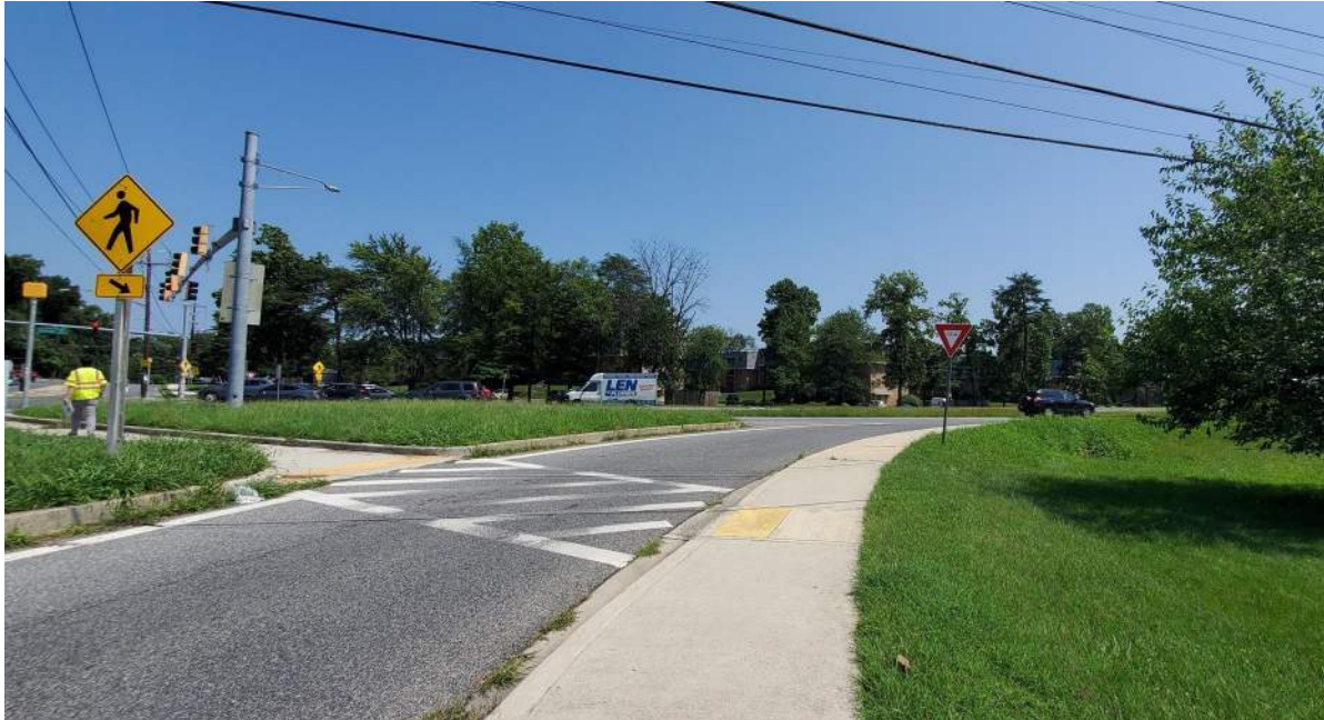
Photo 1.03. Missing pedestrian warning sign assembly – SW corner of Bel Pre Road.
