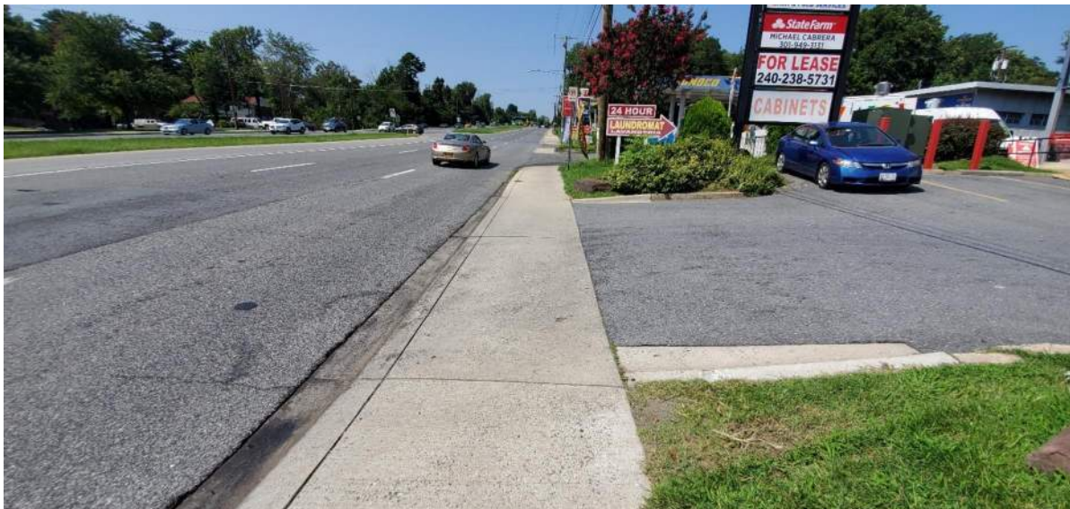
Photo 6.23. Driveway aprons and curb cuts along NB MD 97.
