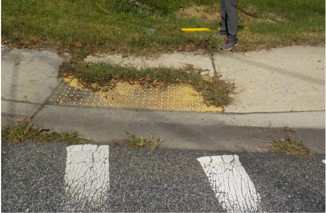
Photo 1.13. Level landing – NW corner of Bel Pre Road.
