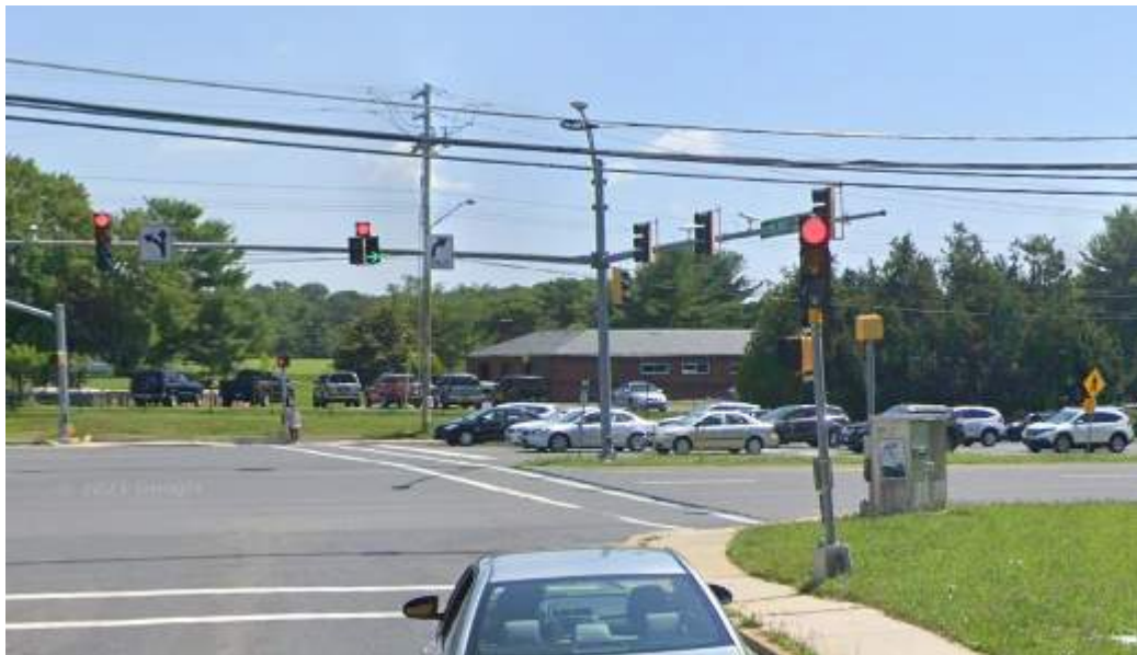
Photo 8.13. Nearside signal head mismatch with mast arm display – Aspen Hill Road approach.
