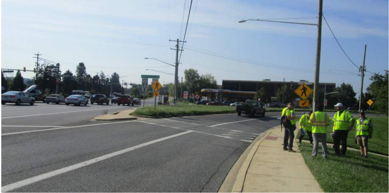
Photo 6.02. Existing warning signs for uncontrolled crossing of dual right turn lane at MD 185.
