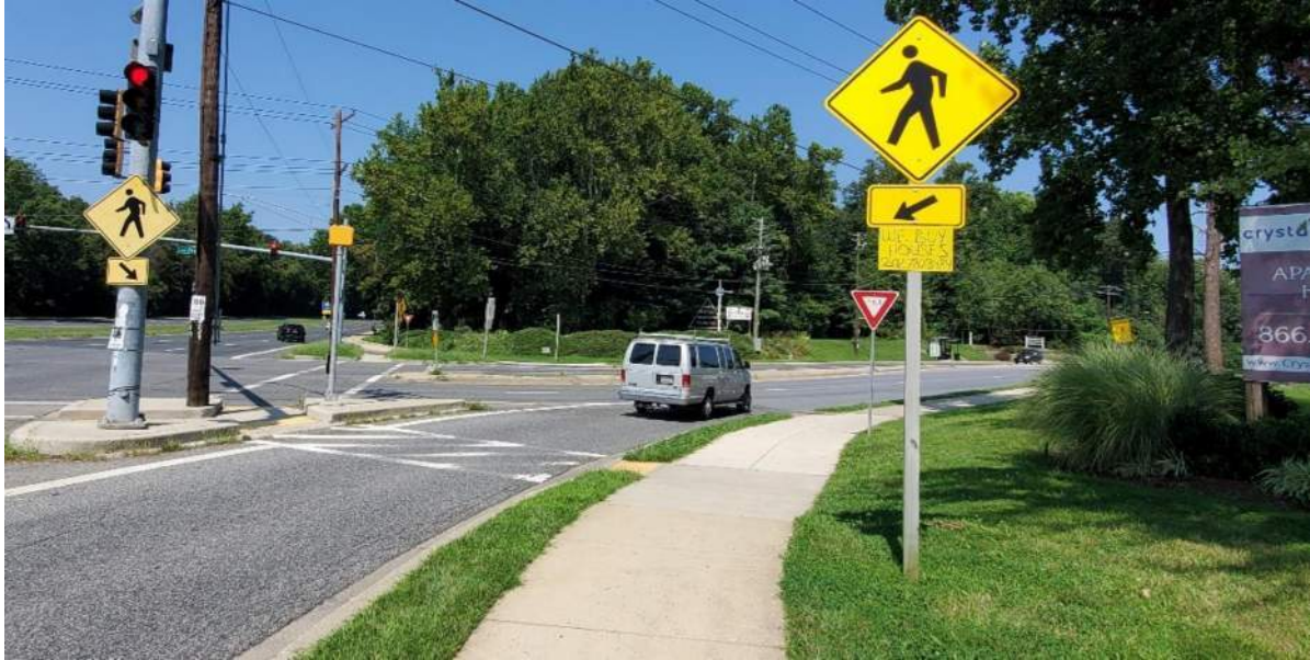
Photo 1.05. Faded warning sign on traffic signal pole – SE corner of Bel Pre Road.
