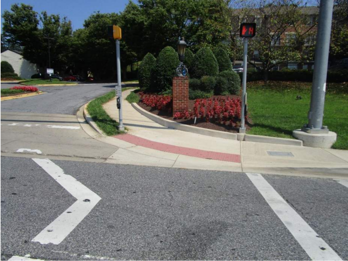
Photo 3.12. Sidewalk running slope – SE corner of Postgate Terrace.
