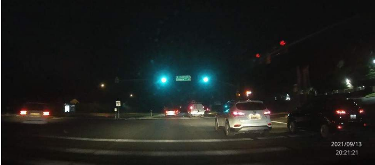
Photo 3.08. No intersection lighting at MD 97 at Heathfield Road / Postgate Terrace.
