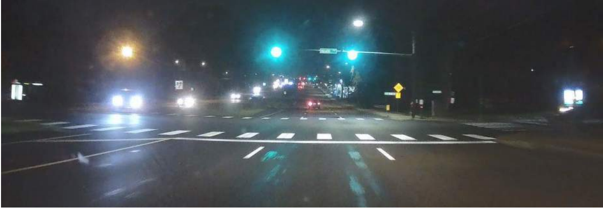
Photo 14.09. NB MD 97 approach to Hewitt Avenue at night.
