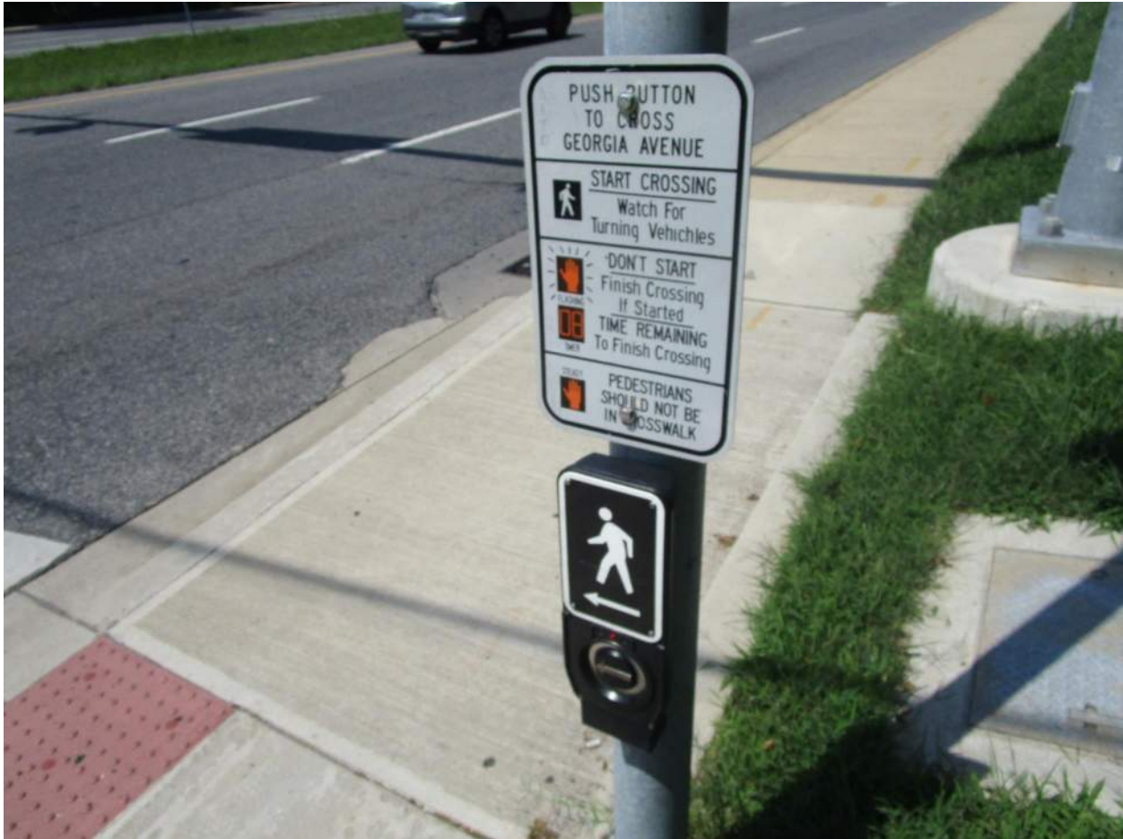
Photo 3.09. APS pushbutton has no audible message – NE corner of Postgate Terrace.
