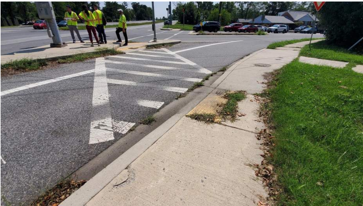
Photo 1.02. Growth and sediment in sidewalk and gutter – NW corner of Bel Pre Road.
