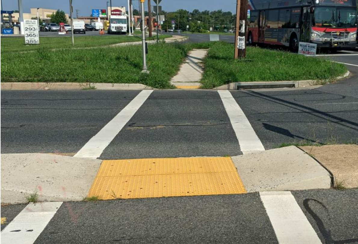
Photo 8.06. Median cut thru – west leg of Aspen Hill Road.
