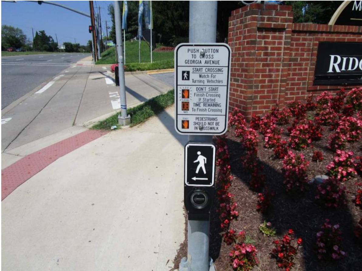
Photo 3.10. APS pushbutton and sign facing away from intersection – SE corner of Postgate Terrace.
