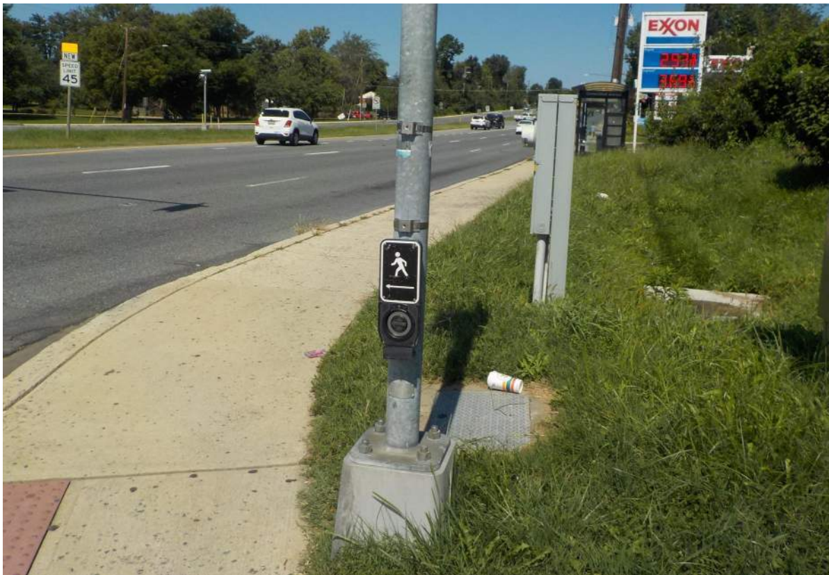
Photo 6.08. Missing pedestrian information sign – NE corner of MD 97 at MD 185.
