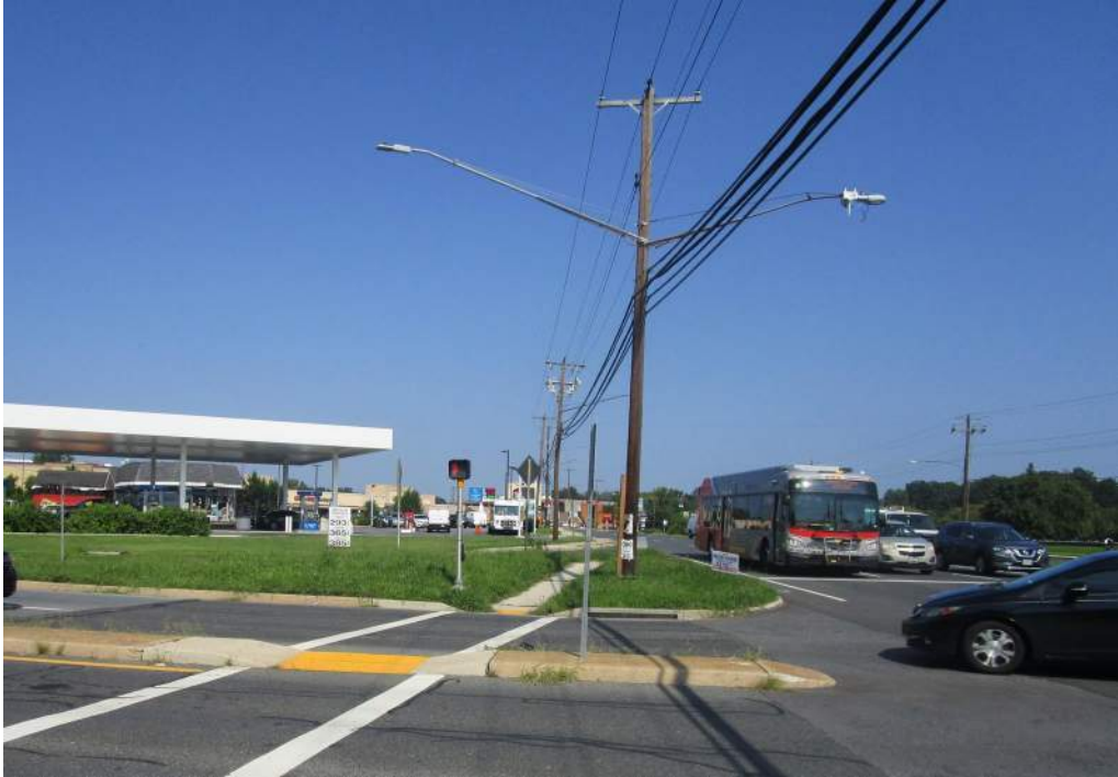
Photo 8.08. Damaged leased light fixture on PEPCO pole – NW corner of Aspen Hill Road.
