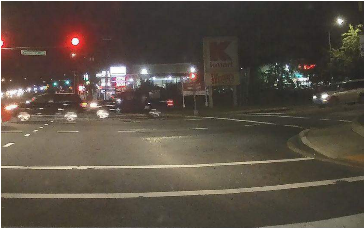
Photo 6.21. Intersection lighting does not cover MD 185 crossings.
