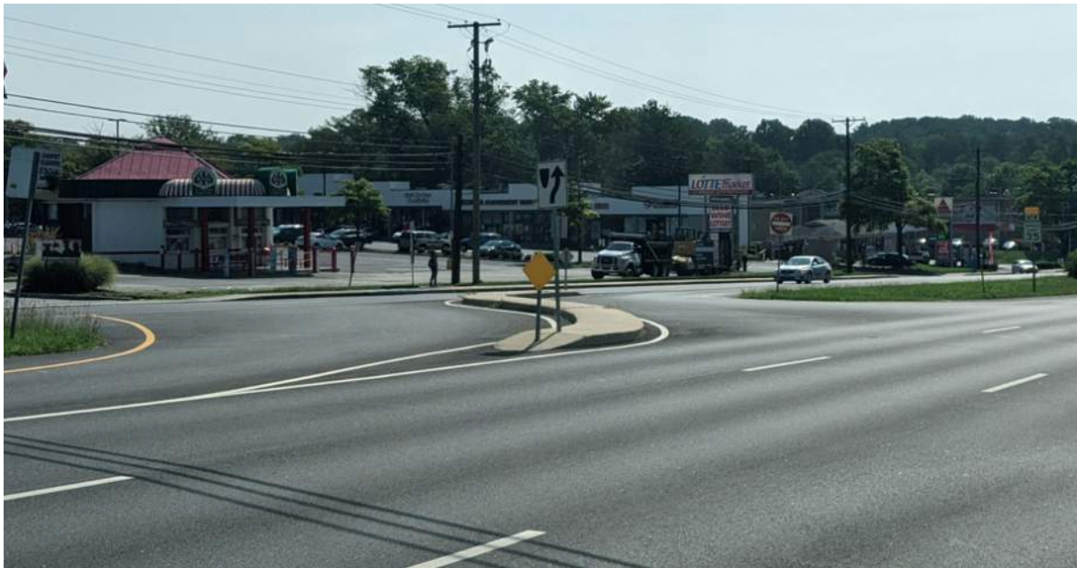
Photo 10.09, 10.11. S-shaped monolithic median in Wendy Lane crossover.
