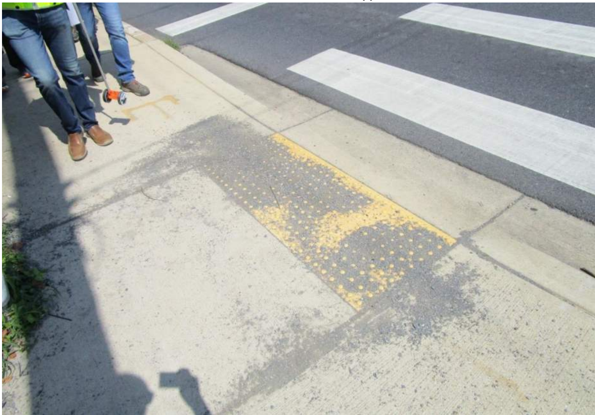
Photo 14.02. Sediment collected in NW level landing for crossing MD 97 at Hewitt Avenue.
