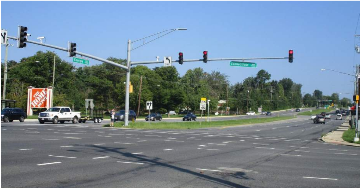
Photo 6.14. Existing traffic signal head displays – NB MD 97 at MD 185.
