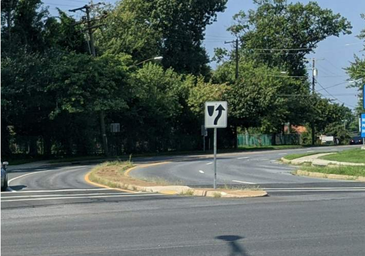
Photo 8.14. Aspen Hill Road median nose missing object marker.
