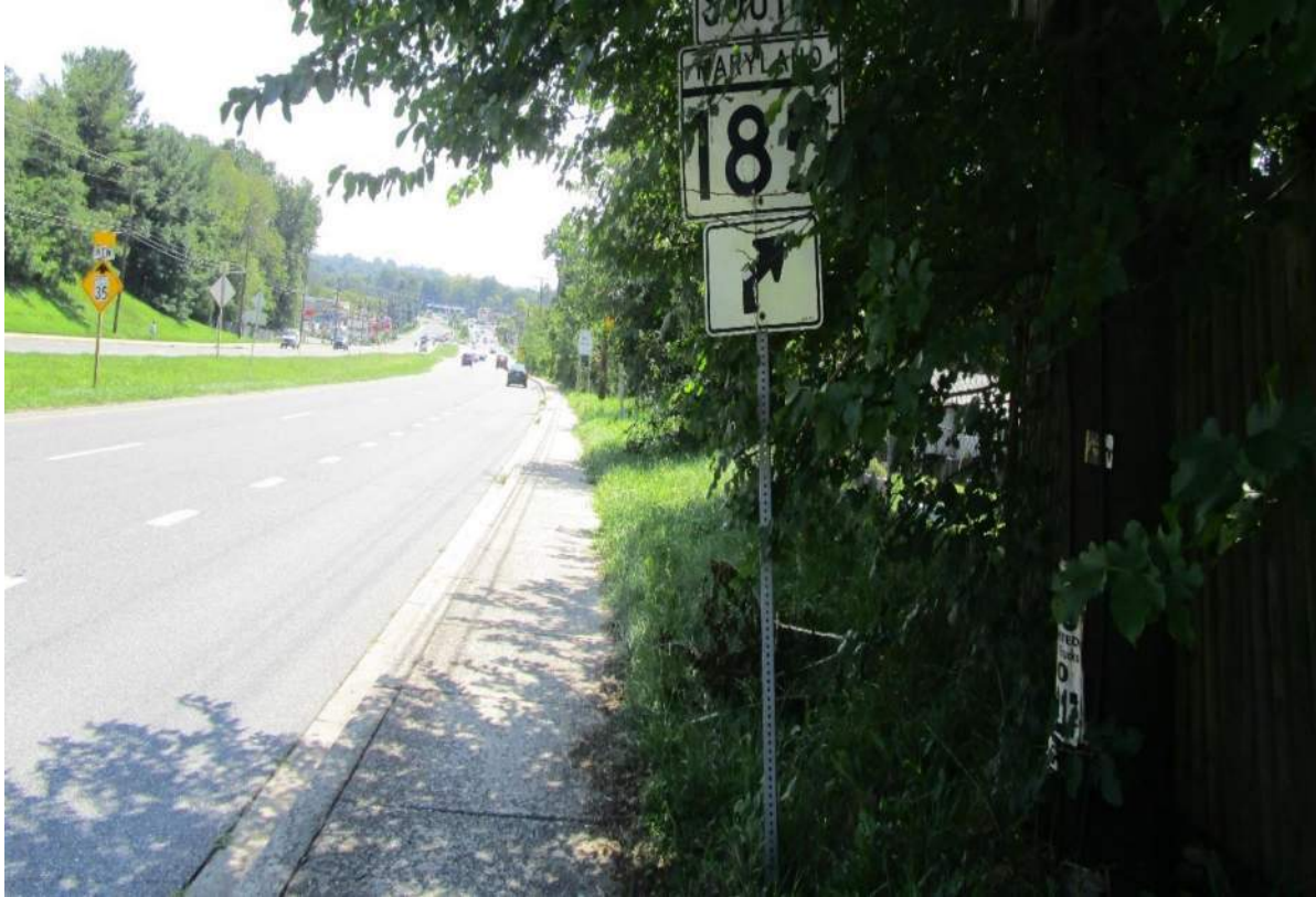
Photo 3.02. Vegetation obstructing sign visibility.
