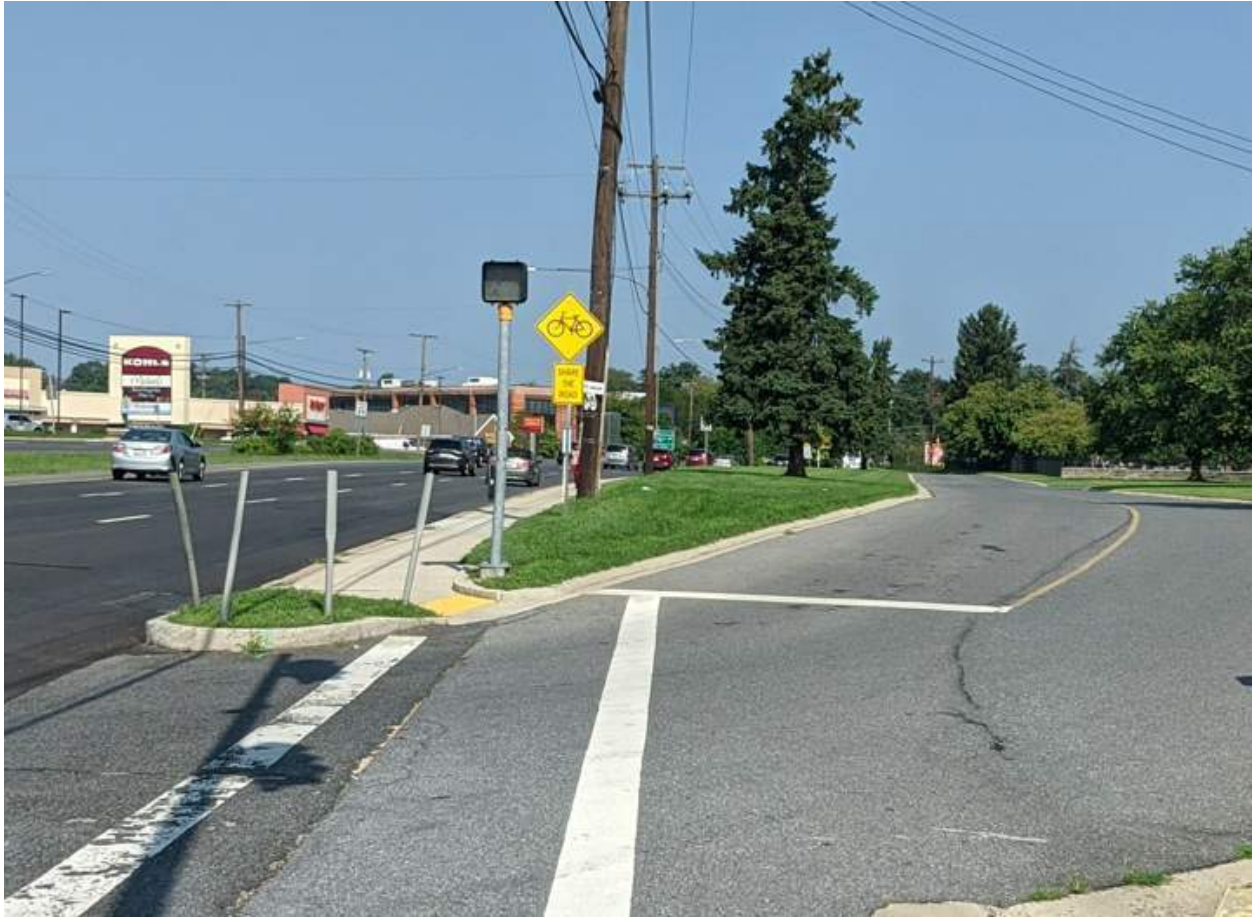
Photo 8.02. Malfunctioning CPS display – Gate of Heaven Cemetery driveway.
