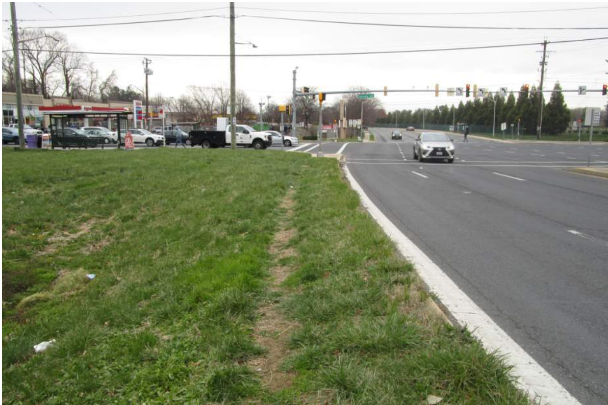
Photo 6.27. "Goat path" along missing sidewalk link in NW corner of MD 185 intersection.
