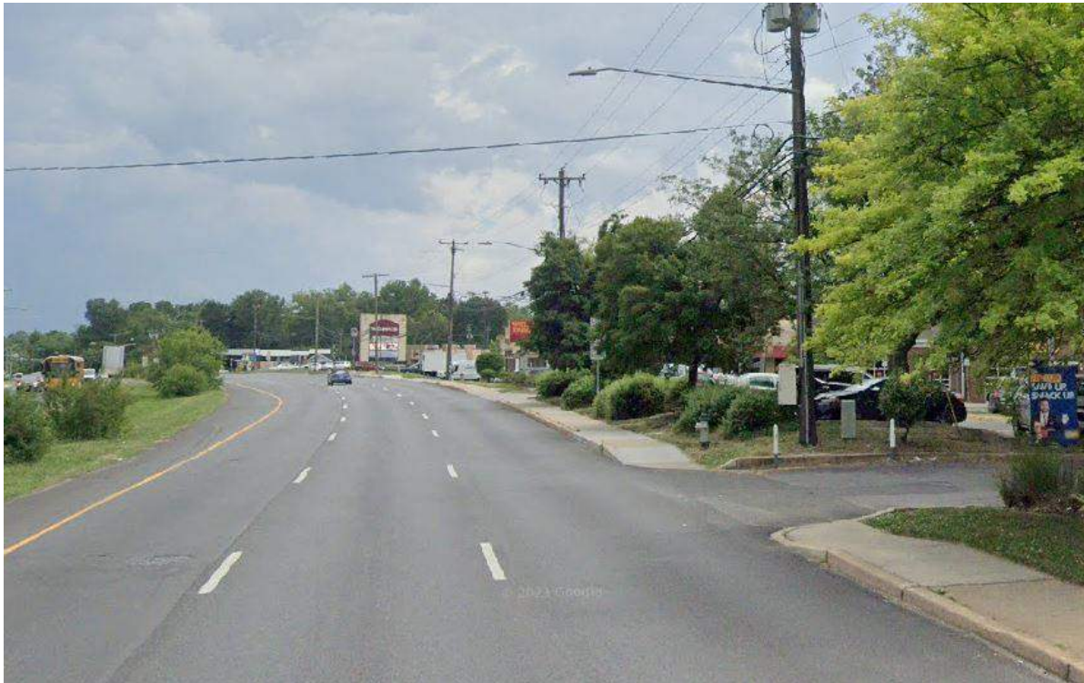
Photo 7.04. Leased light not working (PEPCO #777455-870090).
