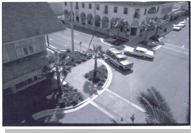
A bulb-out at an intersection reduces the time it takes pedestrians to cross the street, preserves the curb lane for parking, and serves as a traffic-calming device. (Courtesy of Dan Burden, Walkable Communities, Inc.)
