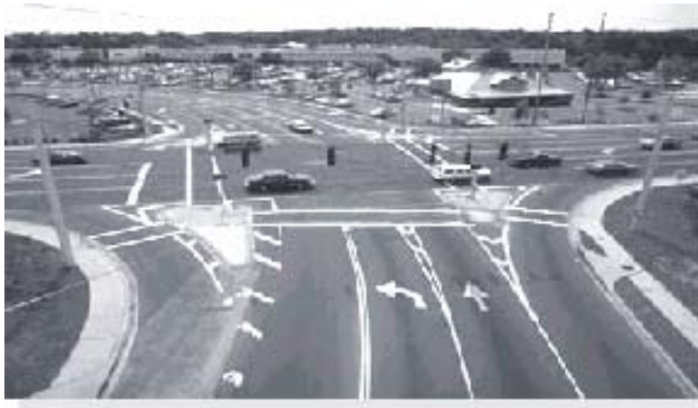
Well-designed slip lanes at a busy, wide intersection. The crosswalks are located to allow the greatest visibility between the drivers and pedestrians.
