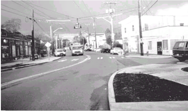
A serpentine street is a curving roadway that encourages slower speeds through the use of curbs and landscaping (Photo by Cara Seiderman)
