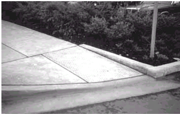
A curb ramp with a single apron incorporates landscaping into the design. (Photo by Peter Lagerwey)
