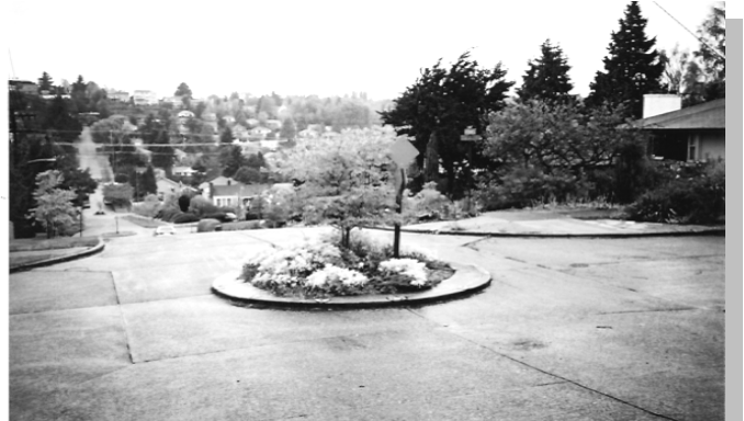
A small traffic circle in the middle of a neighborhood intersection is used as a traffic-calming device.
