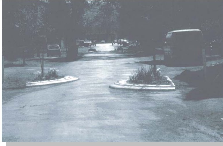
A choker on a two-way roadway narrows the street and serves as a traffic calming device. (Photo courtesy of Dan Burden, Walkable Communities, Inc.)
