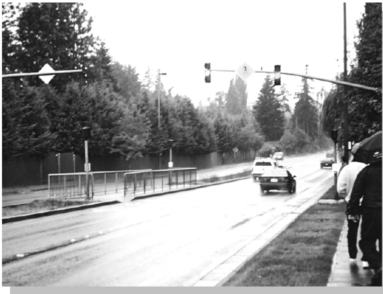
A wide refuge island was installed on the median of a four-lane highway with fencing to channelize pedestrians diagonally across the island so that they see on-coming traffic. Pedestrians have push button traffic control device at their fingertips at both ends of the crosswalk and on the refuge island.
