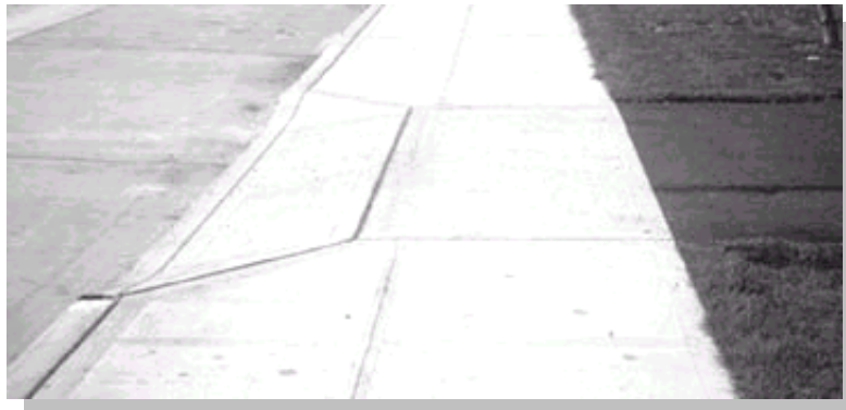
A commercial sidewalk should maintain a continuous, level walkway for pedestrians.
