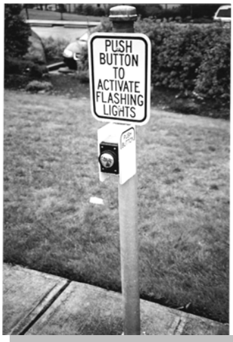
A traffic control button at a crosswalk allows pedestrians to speed up the traffic light cycle so they can cross safely with a signal.
