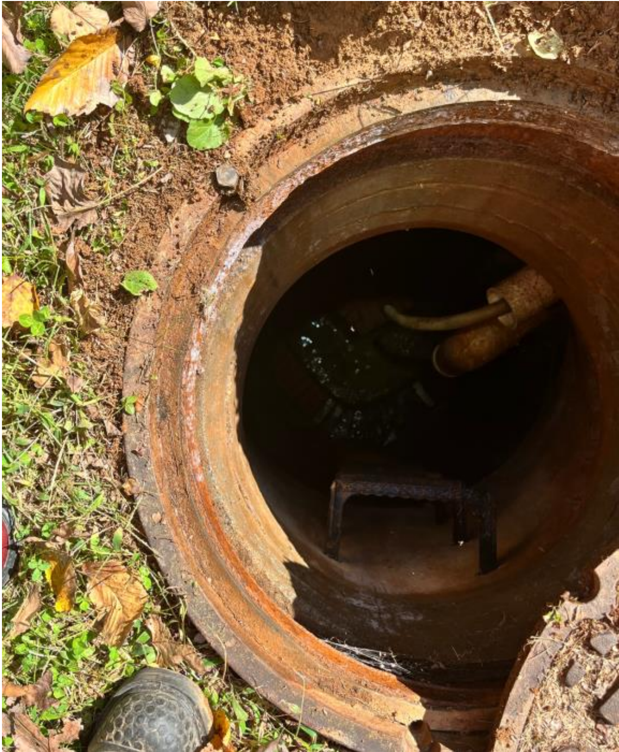
Adjacent Manhole at Hoyles Mill WWPS
