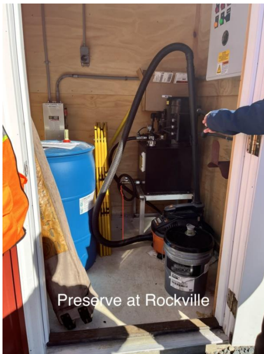
Hourly Chemical injection to sewer flow for F.O.G (Fats, oils and grease) breakdown at Rock Creek WWPS
