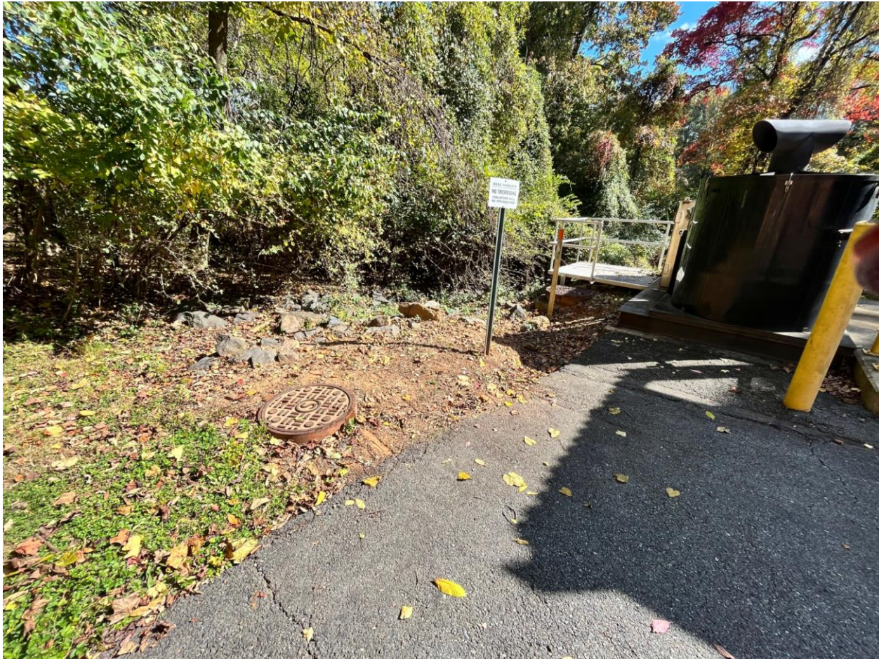
Adjacent Manhole locations at King Farm WWPS.
