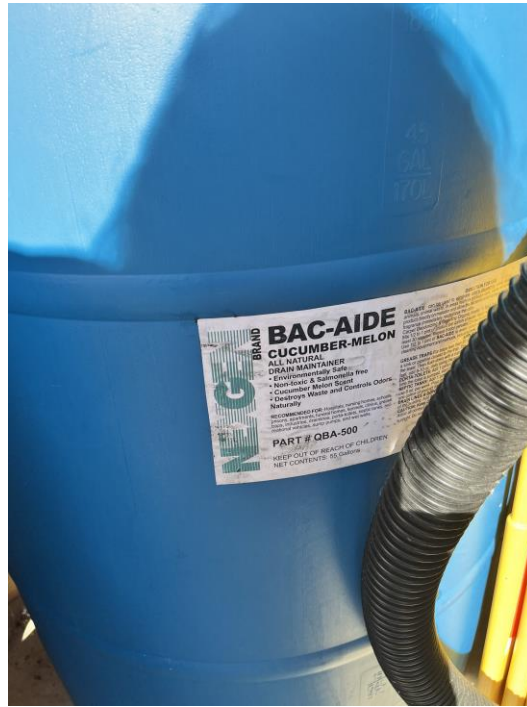
Hourly Chemical injection to sewer flow for F.O.G (Fats, oils and grease) breakdown at Rock Creek WWPS
