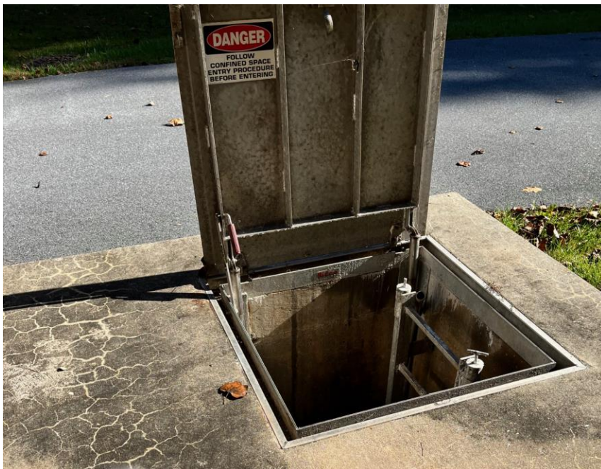
Outside entrance to wet well at Olney WWPS. Approximately 25 ft Deep.
