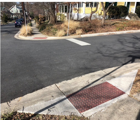
Figure 6-28. An unmarked crossing
