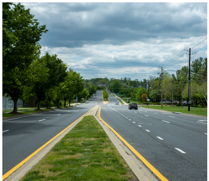
Figure 2-4. MD Route 355 near Cider Mill
