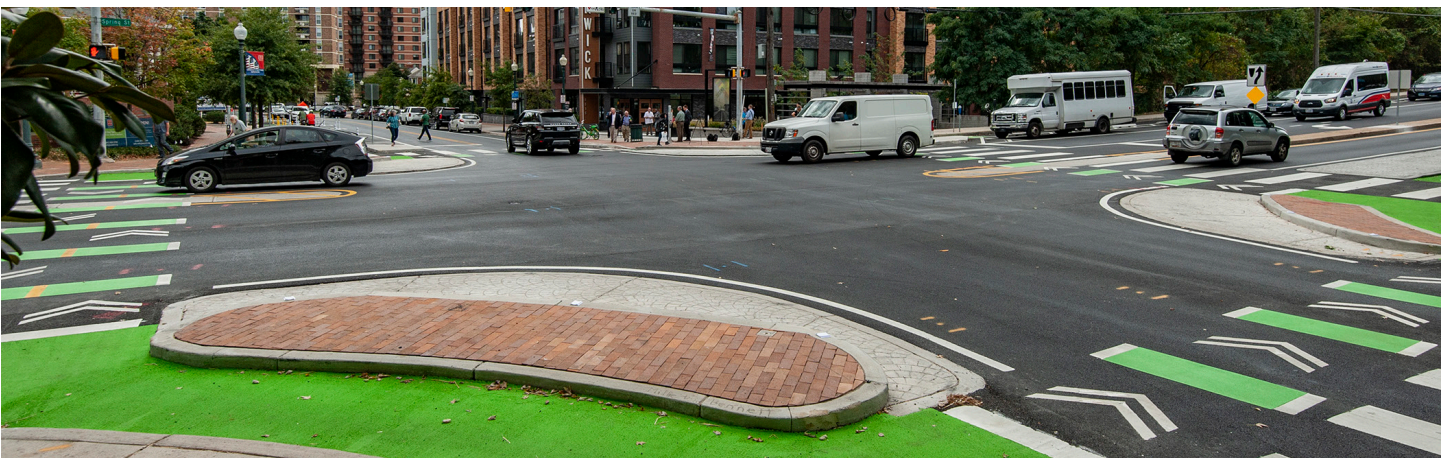
Figure 6-1. A compact intersection at Spring Street and 2nd Avenue in Silver Spring
