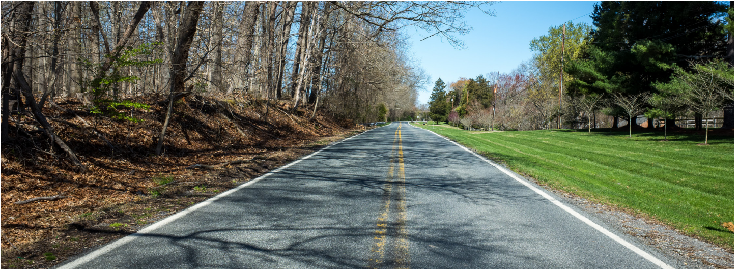
Figure 2-84. Esworthy Road from River Road to Seneca Road
