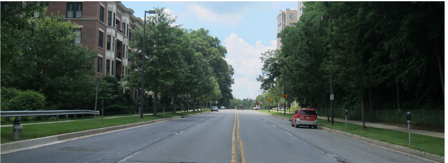
Figure 2-44. Tuckerman Lane near Grosvenor Metro Station
