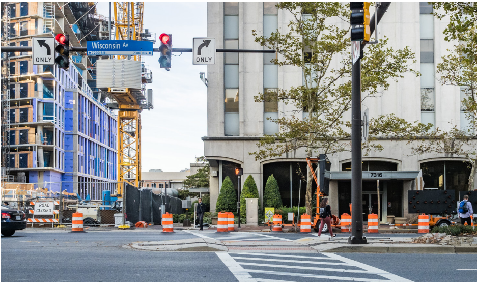
Figure 6-33. The “nose” on top of the median crossing island is key to slowing vehicle speeds and supporting pedestrian comfort.
