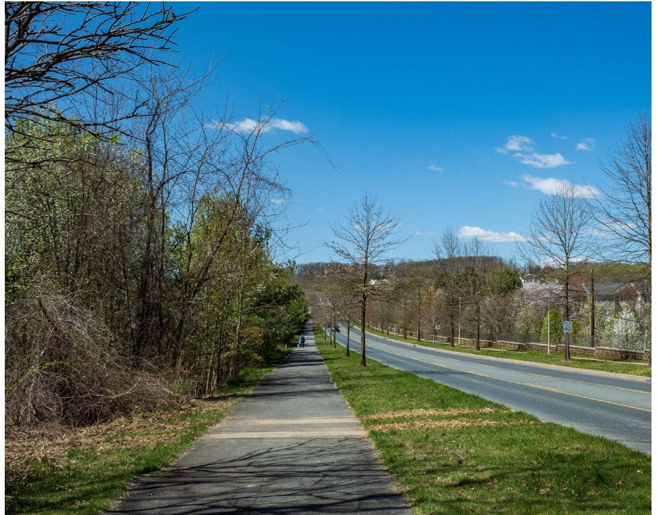
Figure 5-11. Example of a sidepath on Watkins Mill Road
