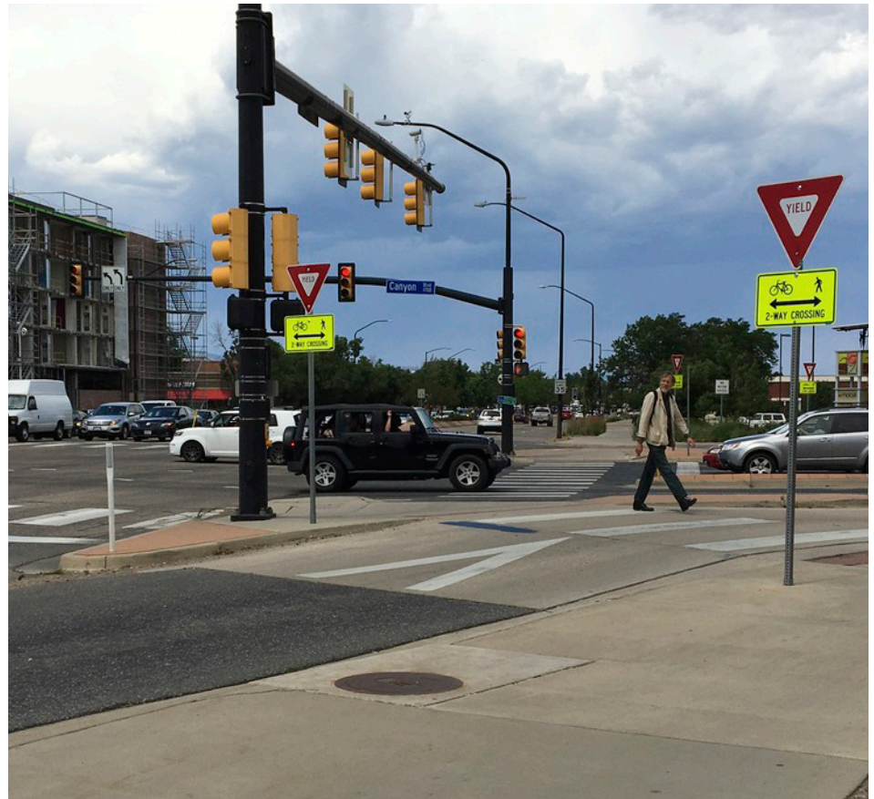
Figure 6-14. A channelized right turn lane with raised crosswalk, high visibility markings and signs
