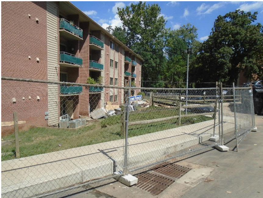
Figure 32 - Top of Inlet Directly in Box Culvert Top Slab
