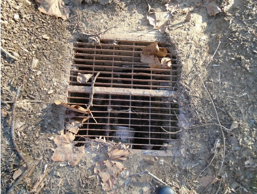
Figure 41 - Inlet with Metal Grate in Depression of Rock Creek Woods Apartments
