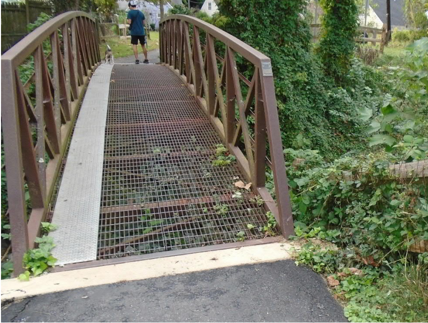
Figure 45 - Pedestrian Bridge over Tributary 1 at Vandergrift Avenue.
