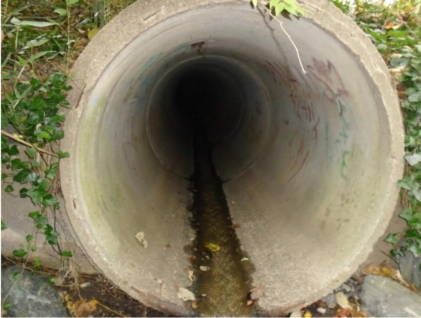
Figure 43 - 60-inch RCP Outfall to Tributary 1.
