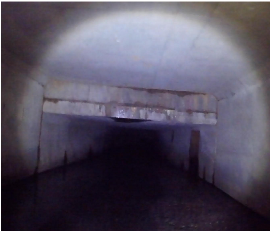
Figure 26 - Inside 14'-0" x 7'-6" Box Culvert Looking Downstream towards 10'-0" x 5'-0" Box Culvert
