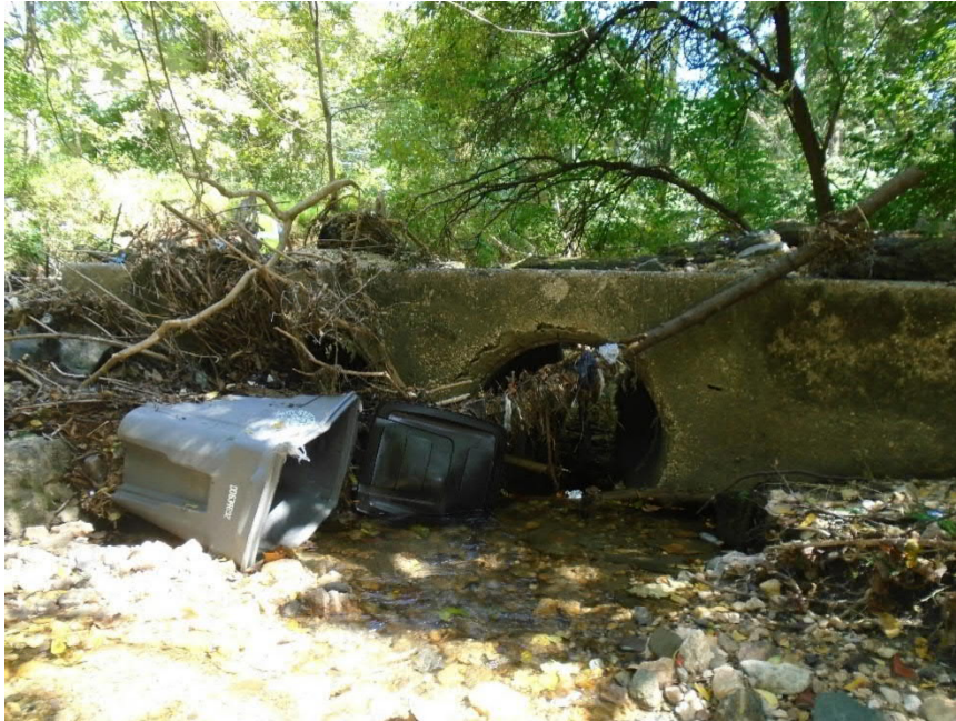
Figure 58 - Abandoned Roadway Culvert Downstream of Culvert Outfall (Photo 1)
