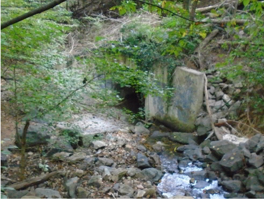
Figure 48 - Headwall of the Tributary 1 Culvert.
