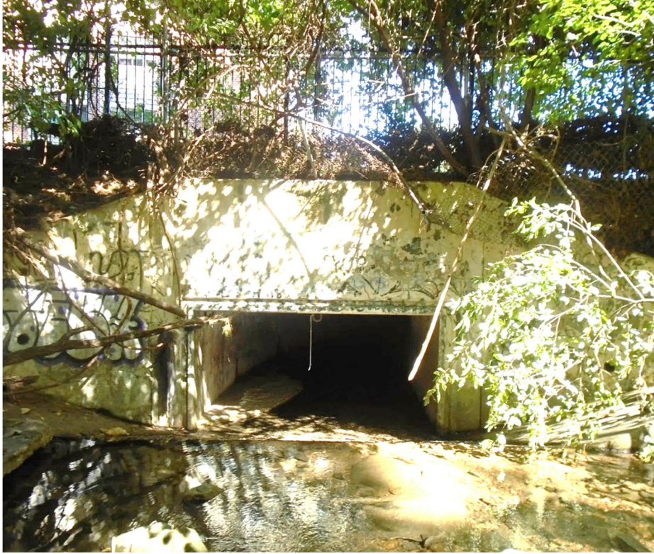
Figure 25 - Northern Culvert, Upstream Headwall
