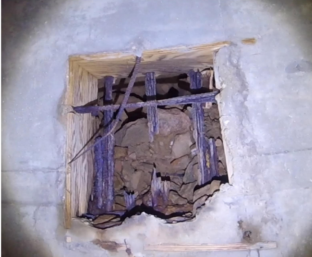
Figure 22 - Blockout in Side Wall of Box Culvert
