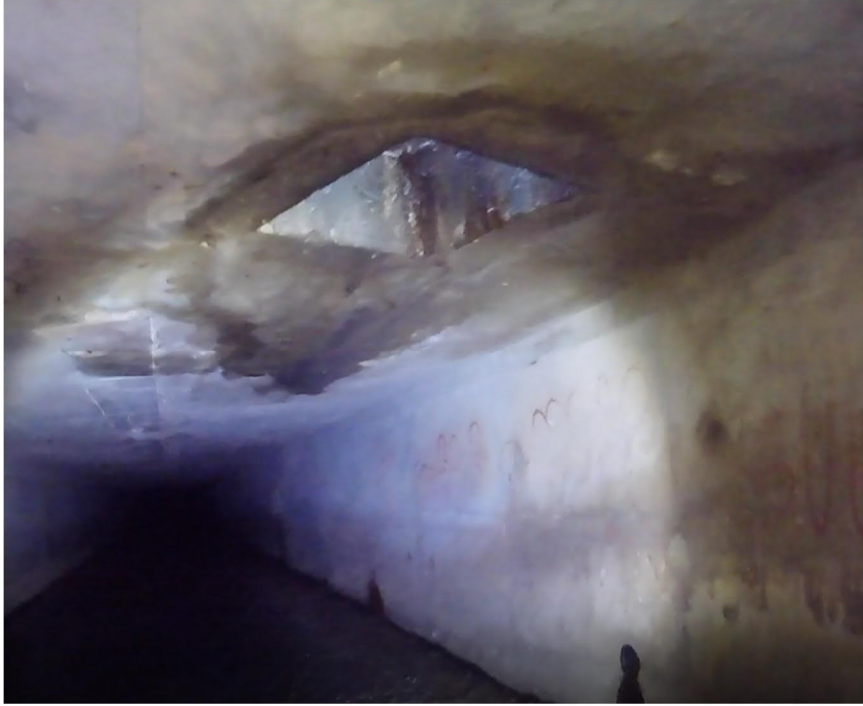
Figure 31 - Underside of Inlet Directly in Box Culvert Top Slab
