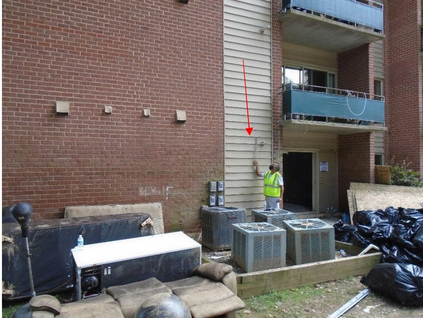
Figure 38 - High Water Mark Building 7
