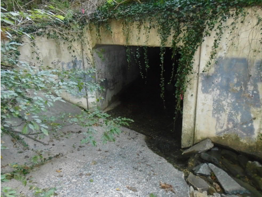
Figure 29 - Southern Culvert Upstream Headwall
