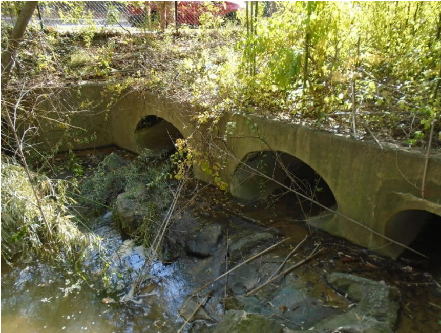
Figure 44 - CMPA Outfall to Tributary 1.
