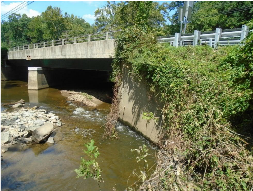
Figure 60 - Veirs Mill Road Over Rock Creek.
