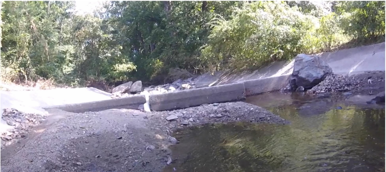
Figure 28 - Downstream Velocity Dissipators
