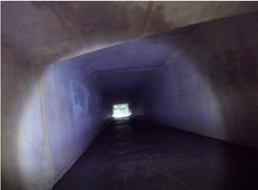
Figure 30 - Inside 10'-0" x 5'-0" Box Culvert Looking Upstream towards 10'-0" x 8'-6" Box Culvert
