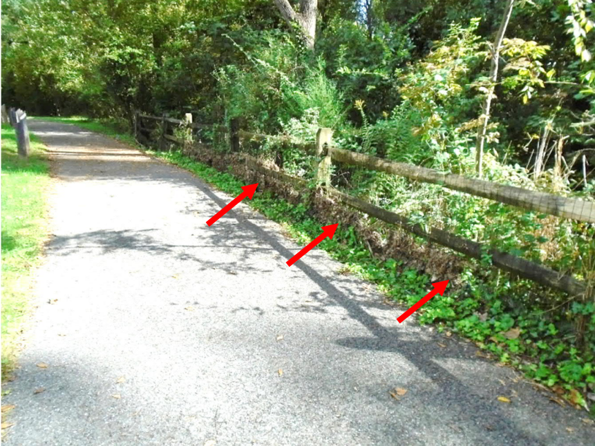
Figure 55 - Debris in Fence Adjacent to Tributary 2.
