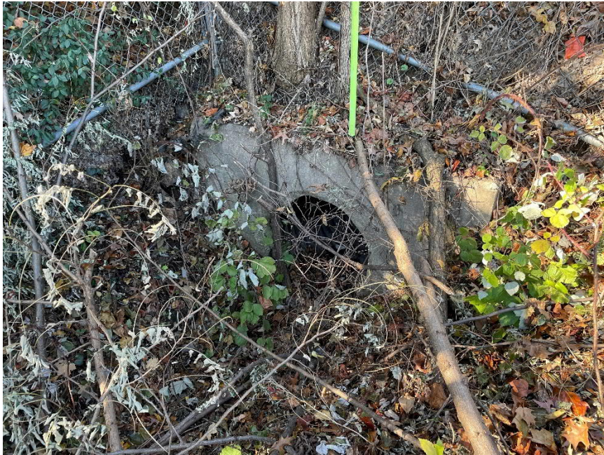
Figure 69 - Upstream storm drain outfall at concrete flume.
