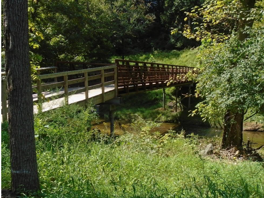
Figure 61 - Pedestrian Bridge Crossing Downstream of Viers Mill Road Bridge.
