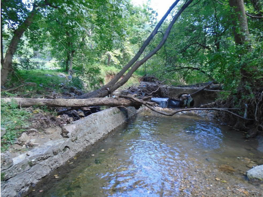
Figure 59 - Abandoned Roadway Culvert Downstream of Culvert Outfall (Photo 2).
