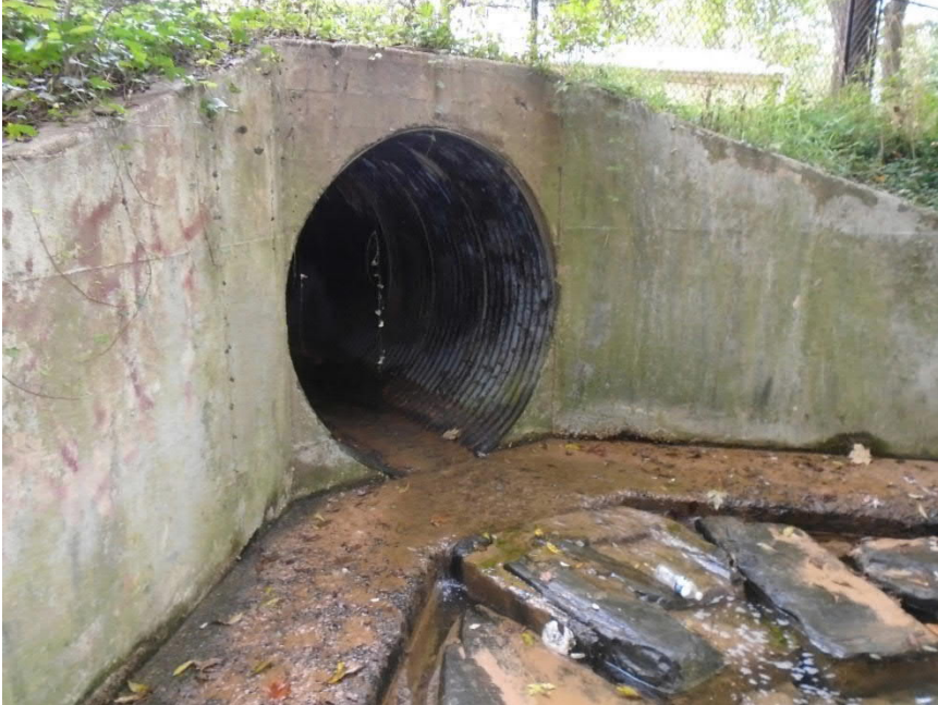
Figure 50 - 66-inch CMP Outfall to Tributary 2.
