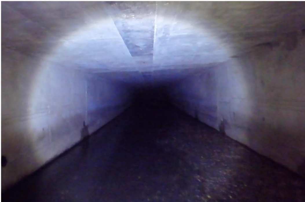
Figure 21 - Typical View inside of Box Culverts.
