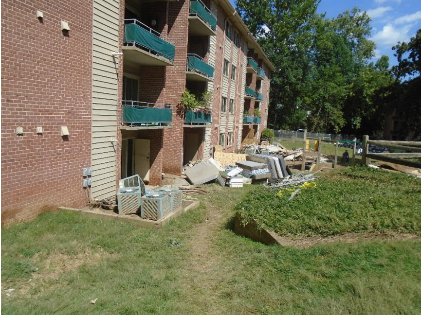
Figure 34 - Area of Flooding and Debris Clean Up
