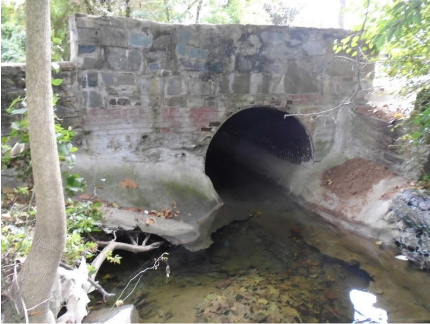
Figure 46 - Tributary 1 CMPA Crossing South of the Twinbrook Community Recreation Center.
