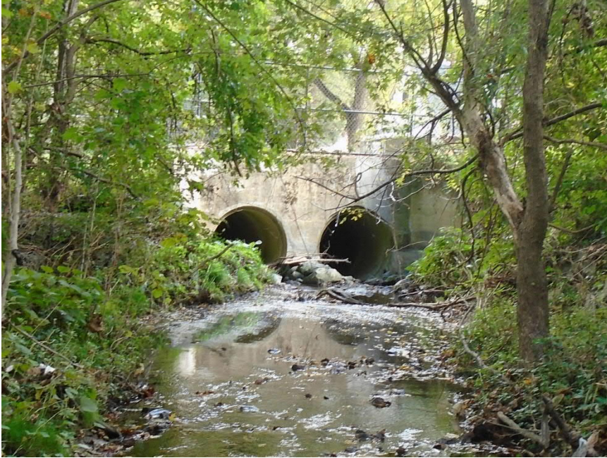
Figure 52 - Ardennes Avenue Crossing Tributary 2.
