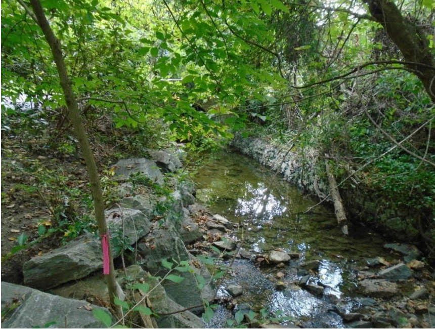
Figure 42 - Typical stream and bank conditions of Tributary 1.
