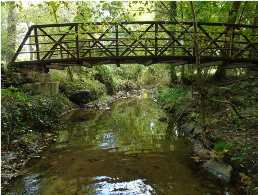
Figure 51 - Pedestrian Bridge Crossing Tributary 2 Downstream of Outfall.
