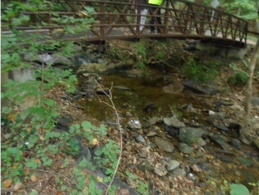
Figure 47 - Pedestrian Bridge Crossing Tributary 1 North of the Twinbrook Community Recreation Center.
