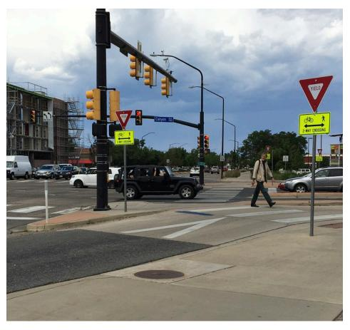
Figure 6-14. A channelized right turn lane with raised crosswalk, high visibility markings and signs
