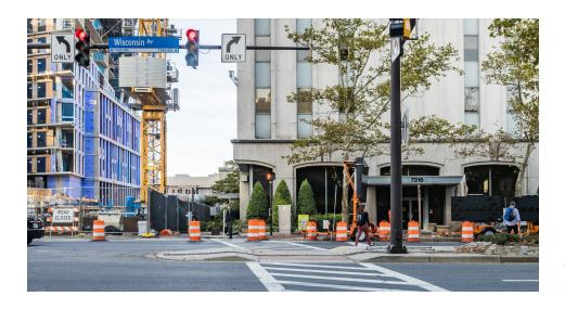
Figure 6-32. The "nose" on top of the median crossing island is key to slowing vehicle speeds and supporting pedestrian comfort.
