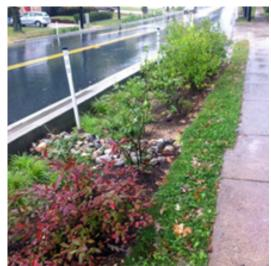
Figure 7-7: Examples of rain gardens (Source: Montgomery County Department of Environmental Protection)
