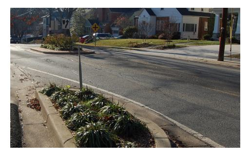
Figure 9-8: Horizontal traffic calming treatment
