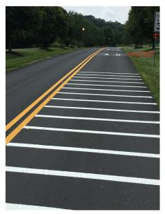
Figure 9-11. Example of optical speed bars
