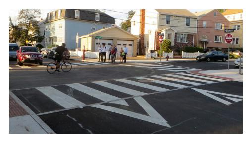
Figure 6-33. Image of a raised intersection
