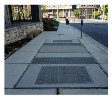
Figure 4-13. Example of grates that may present tripping hazards
