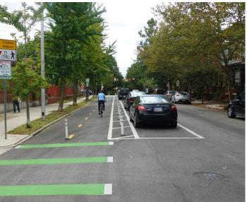
Figure 8-5: Examples of types of separation for separated bikeways
