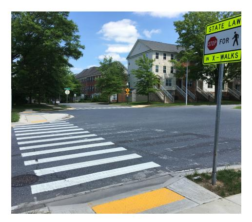
Figure 6-18. Street corner with two perpendicular curb ramps that align with crosswalks
