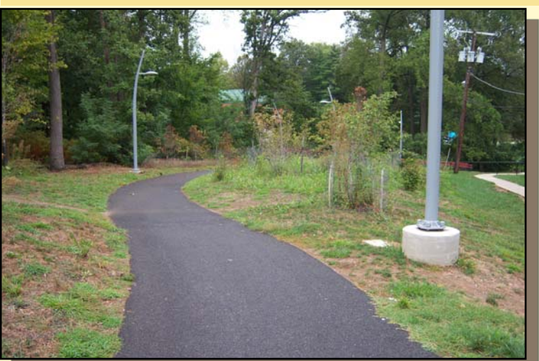
Example of paved off trail road.
