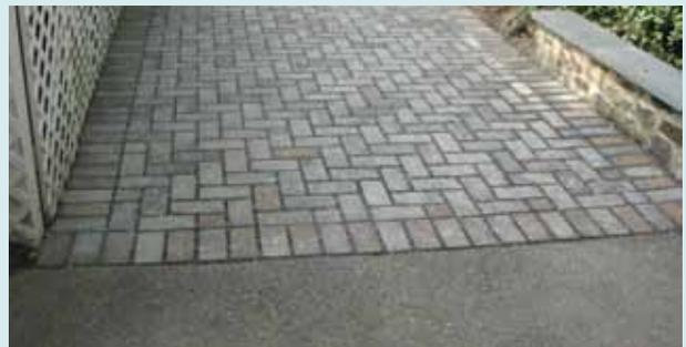
Driveway showing transition from impermeable to permeable
