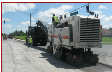
Typical milling (pavement excavating) operation.
