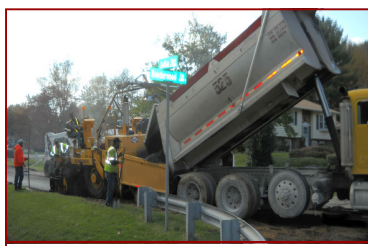
Typical asphalt paving operation.
