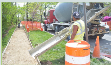
New concrete is poured into forms
