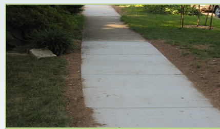
Completed sidewalk repair
