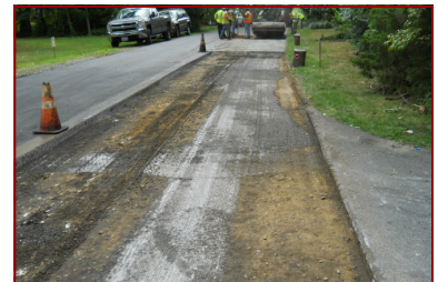
Pavement will be replaced in 2 phases
