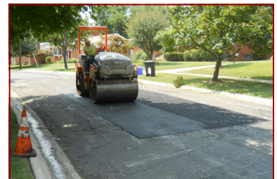
New asphalt is placed and compacted
