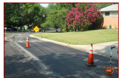
New patch is flush with existing pavement
