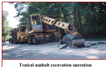
Typical asphalt excavation operation
