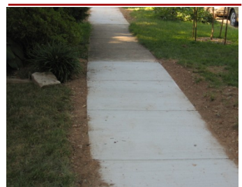
Completed sidewalk repair
