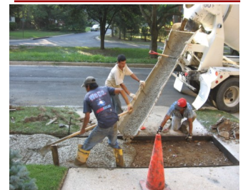
New concrete is poured into forms
