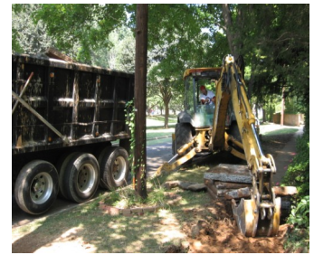
Defective concrete is removed
