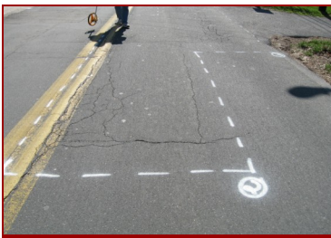
Typical paint markings.
