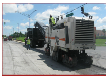
Typical milling operation
