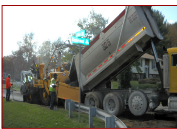
Typical asphalt paving operation
