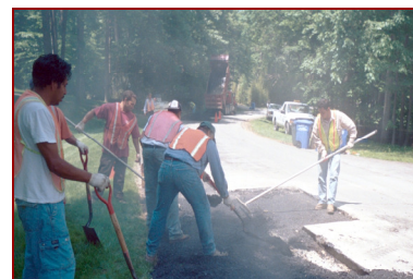
Compacting the sub-grade
