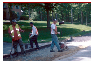
New asphalt is placed and compacted
