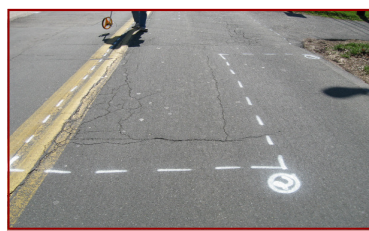
Typical patching paint markings
