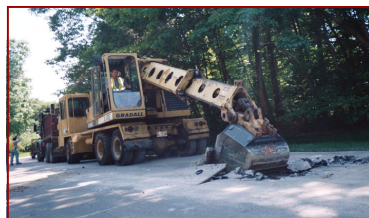
Typical asphalt excavation operation
