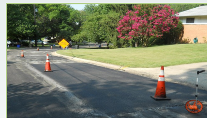
New patch is flush with existing pavement
