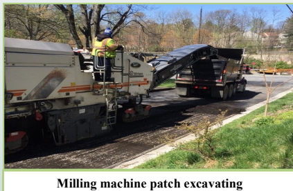
Milling machine patch excavating
