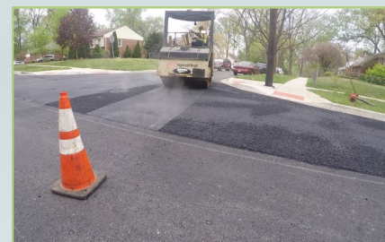
New asphalt is placed and compacted
