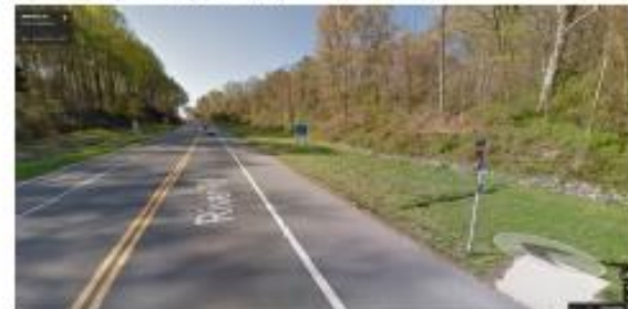
VIEW LOOKING WEST ON RIVER ROAD AT INTERSECTION WITH BRIDGE
