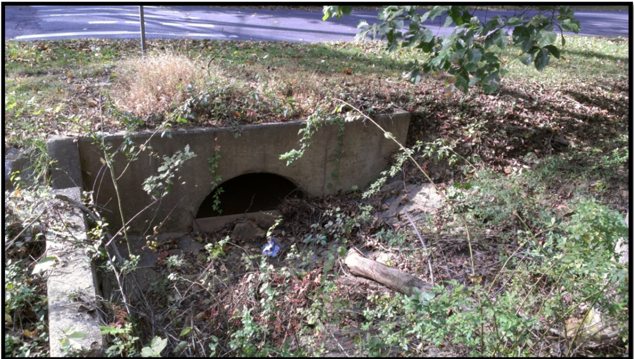
FIGURE 2: Sycamore Culvert Headwall
