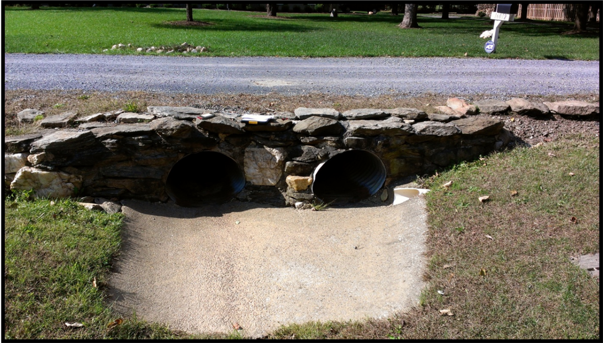
FIGURE 5: Willow Culvert Headwall
