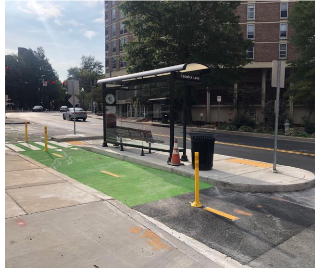
Multiple changes along a stretch of roadway
