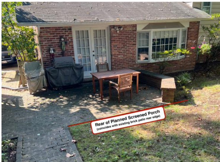
Photo #3: This photo shows the back side of the house where the planned screened porch will be attached. It will essentially be placed on the same footprint as the existing brick patio which is located 16-feet from the rear property line. Another reason for this location is the existing French Doors which will naturally lead into the screened porch from the house.
