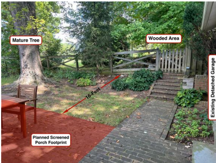
Photo #2: This photo shows another angle that includes the mature Silver Maple tree to the left in relation to the planned screened porch footprint. The presence of the tree further limits building options in the rear yard. The planned screened porch sits nicely on the footprint of the existing brick patio.
