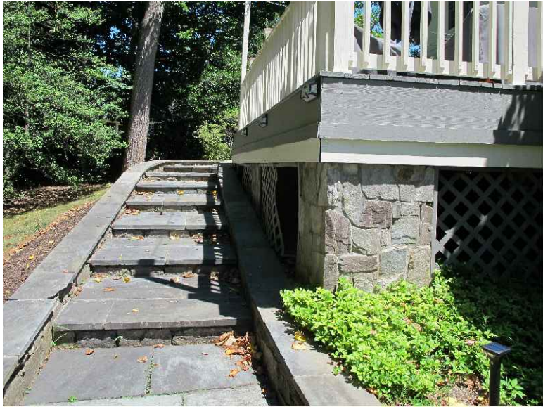
VIEW OF EXISTING STAIRS
