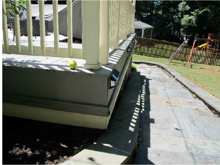
VIEW OF EXISTING STAIRS DOWN TO DRIVEWAY
