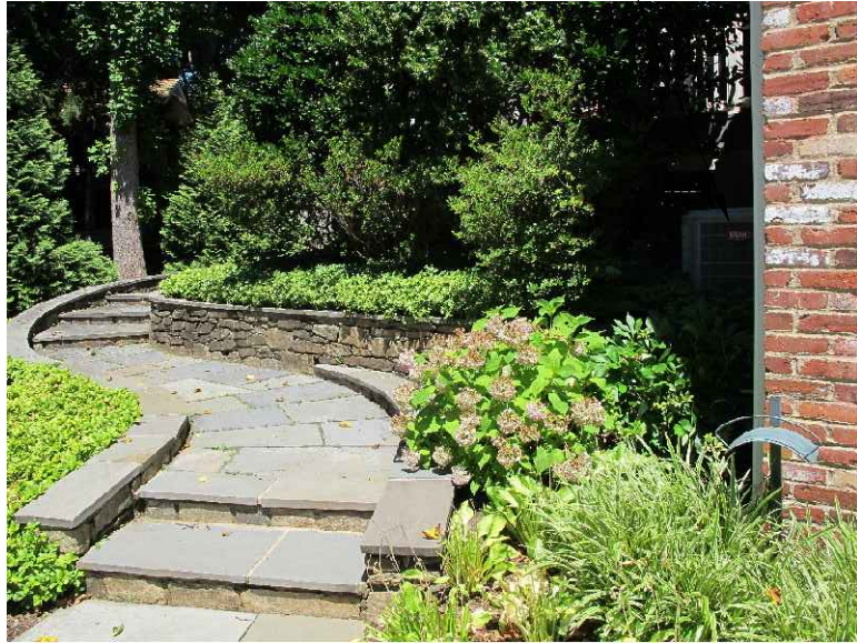
VIEW OF EXISTING STAIRS AND RETAINING WALLS
