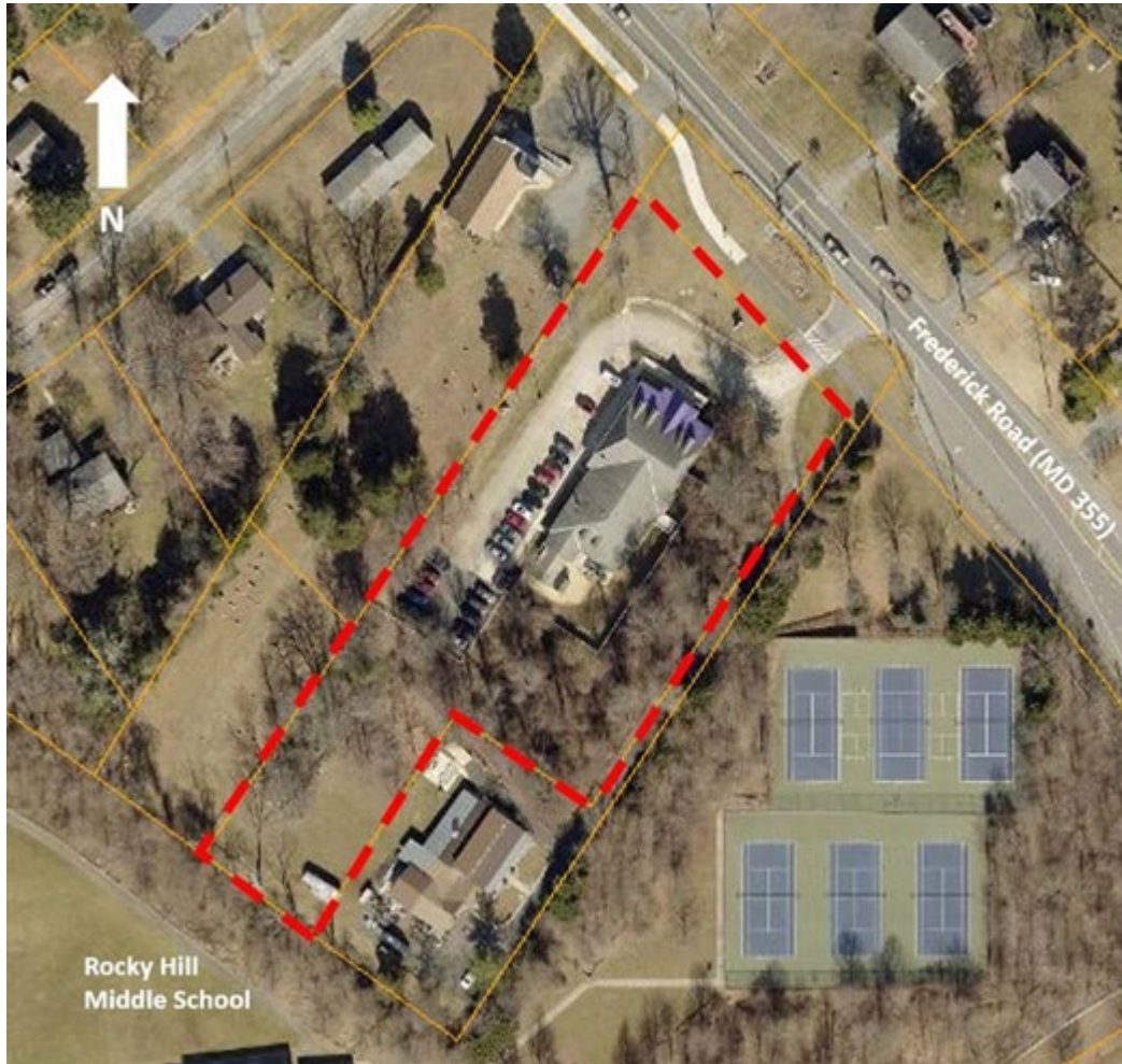
Staff Report - Exhibit 28 Figure 2 – Subject Property
