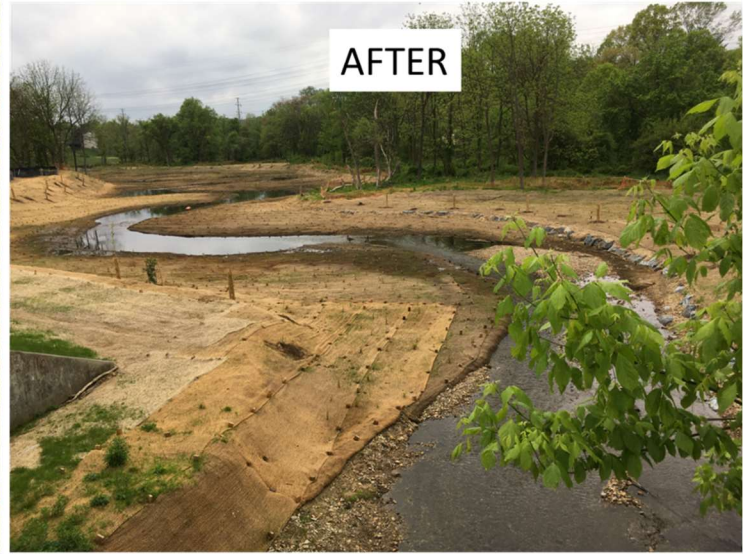
(Stream "restoration" in Blohm Park, Gaithersburg at Watkins Mill Rd. over Whetstone Run at the same location. Note the stream bank armor-plating on the right. (Left on 9/3/2020; right on 5/03/2021); by K.Bawer)
