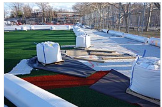
Artificial turf being installed on a baseball field in Queens, New York City.
