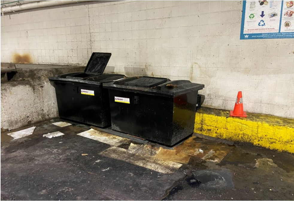
Figure A-3. Grease Spills and Poorly Maintained Used Grease Containers
