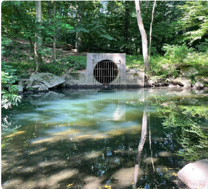
Storm drain outfall inspected in 2024
