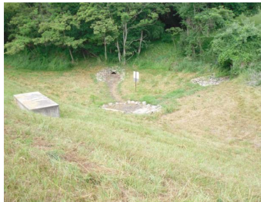
Creating Permanent Pool at Inflow to Pond
