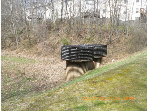
Existing corrugated metal riser
