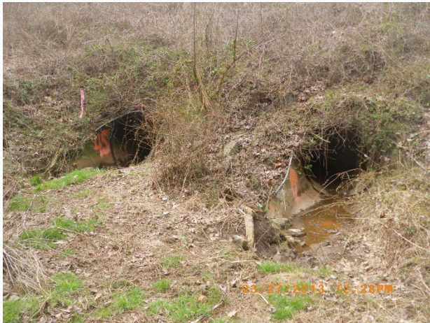
Existing pond outfall pipes
