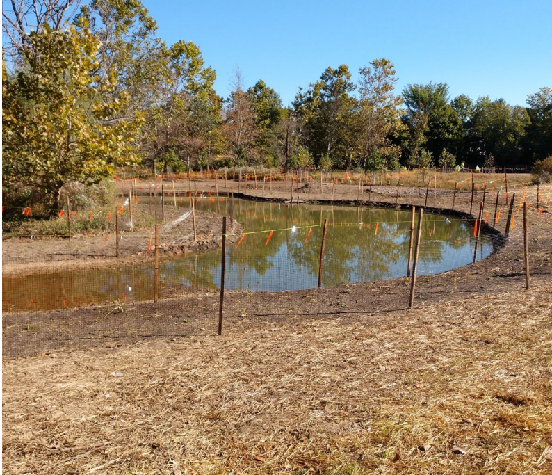
Immediately after construction
