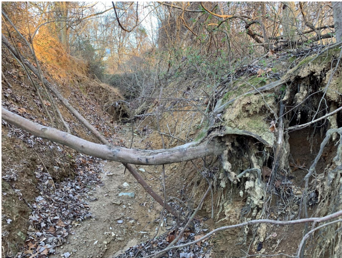
Photo 4: Middle of Erosion Channel
