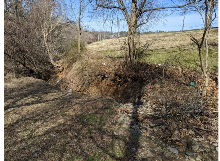
Photo 3: Upstream limits of Erosion Channel
