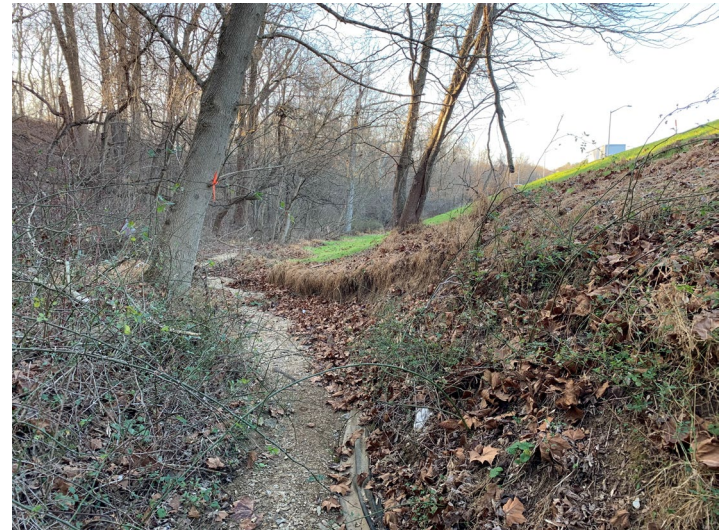
Photo 5: Downstream limits of Eroded Channel
