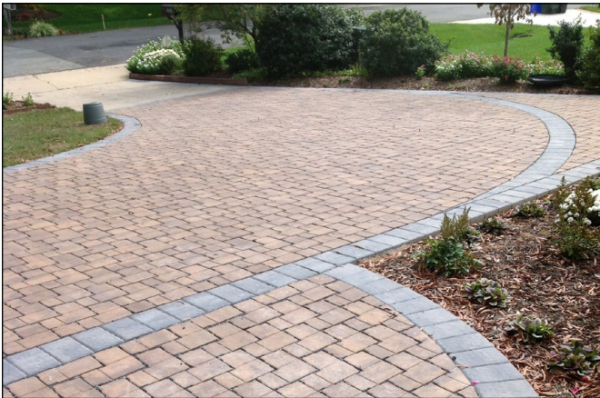
Permeable interlocking paver driveway.
