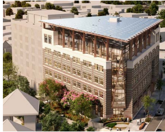
Figure 1: The American Geophysical Union building in Washington, DC underwent a major renovation enabling it to reach high levels of performance. The project achieved net zero energy status using LEED as a guide and tool.
