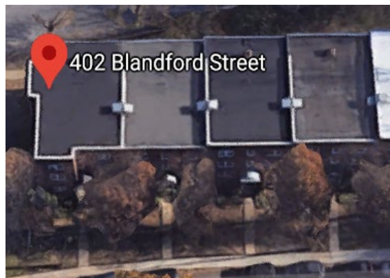
Townhomes with no shared systems or interior area
