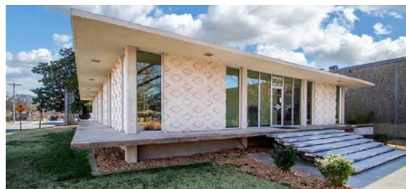
Figure 2: Entegri headquarters in Little Rock, Arkansas was the first LEED Zero building in the United States.
