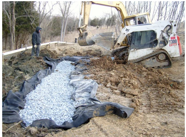
Photo 7 – Infiltration Trench Installation (during repairs)
