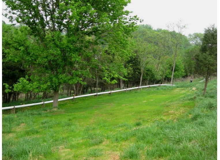
Photo 9 – Area of Leachate Seep (after repairs)
