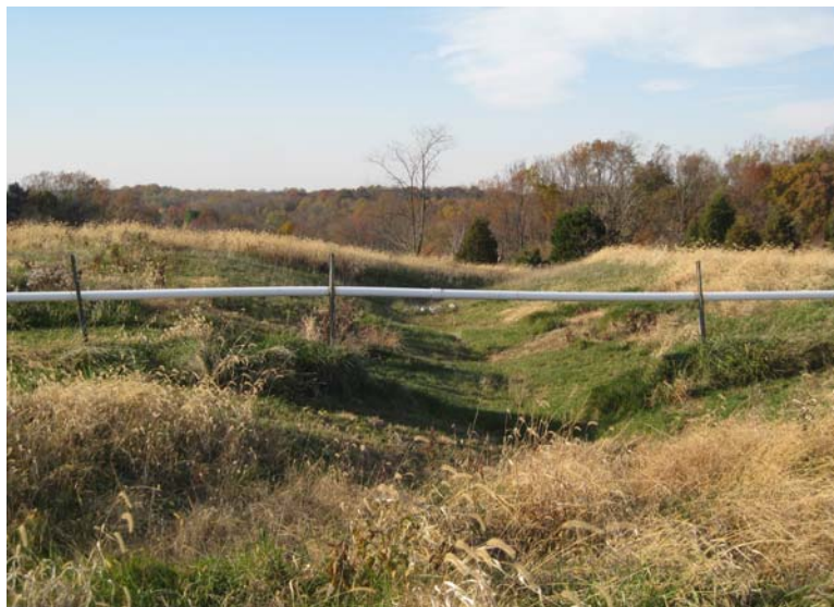
Photo 3 – Drainage Channel (after repairs)
