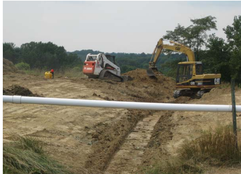
Photo 2 – Drainage Channel Installation (during repairs)
