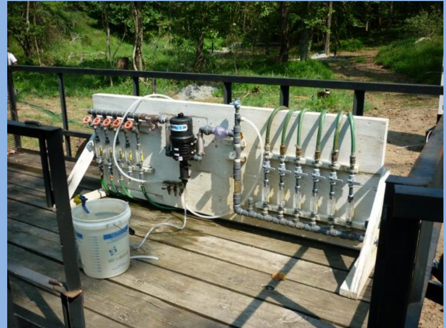
Manifold for injecting EVO/water
