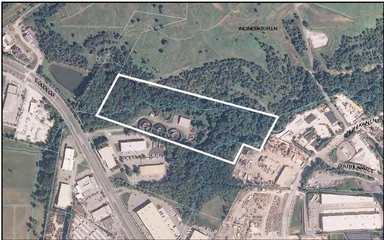
Figure 2 Existing Abandoned WWTP at Gude Drive
