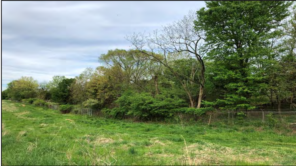
Photo 7 – Gude Landfill Northwest Slope
