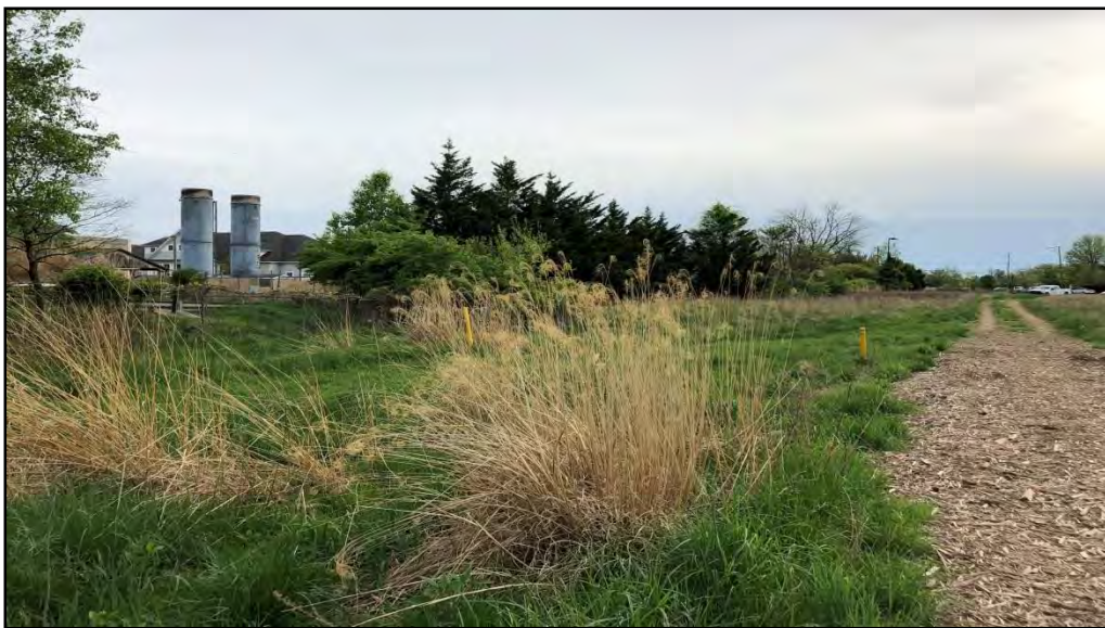
Photo 2 – Gude Trail with view of Flare Station
