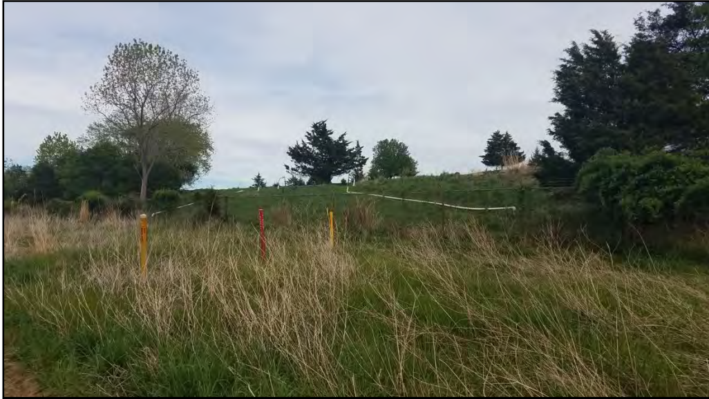
Photo 5 – Gude Landfill Northwest Slope
