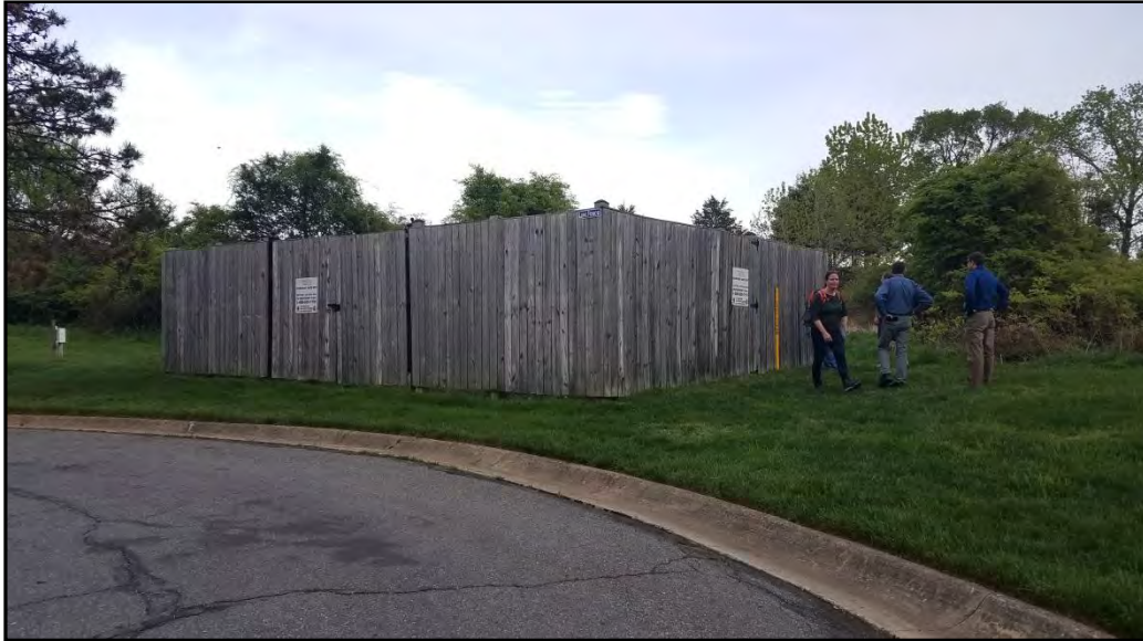
Photo 17 – Columbia Gas Equipment Shelter at Dubuque Court
