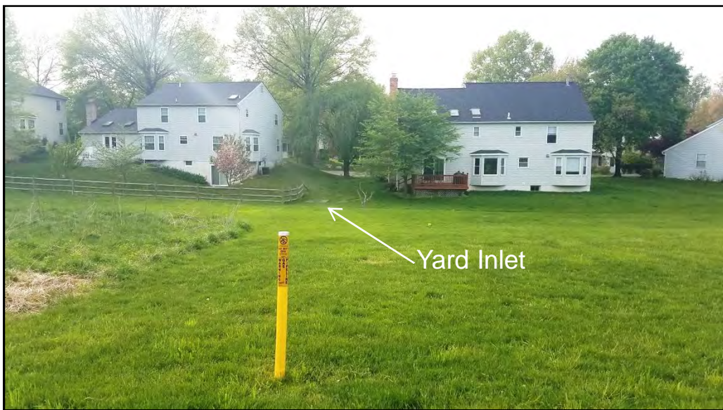
Photo 10 – Existing Yard Inlet adjacent to Derwood Station South properties, Gude Trail, and Columbia Gas/Williams Gas Rights-of-Way (no vegetative screening)
