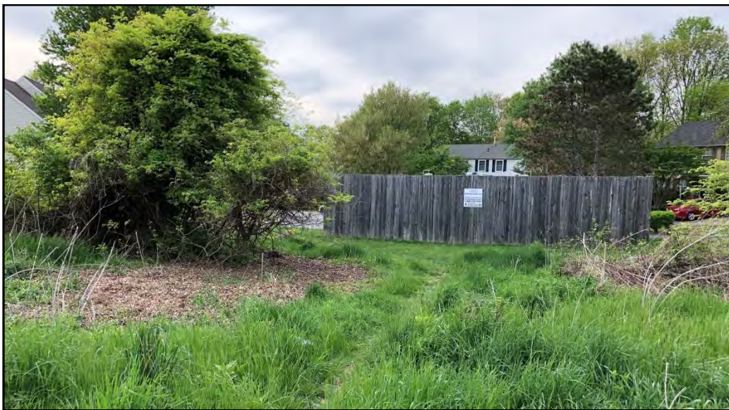
Photo 18 – Columbia Gas Equipment Shelter at Dubuque Court
