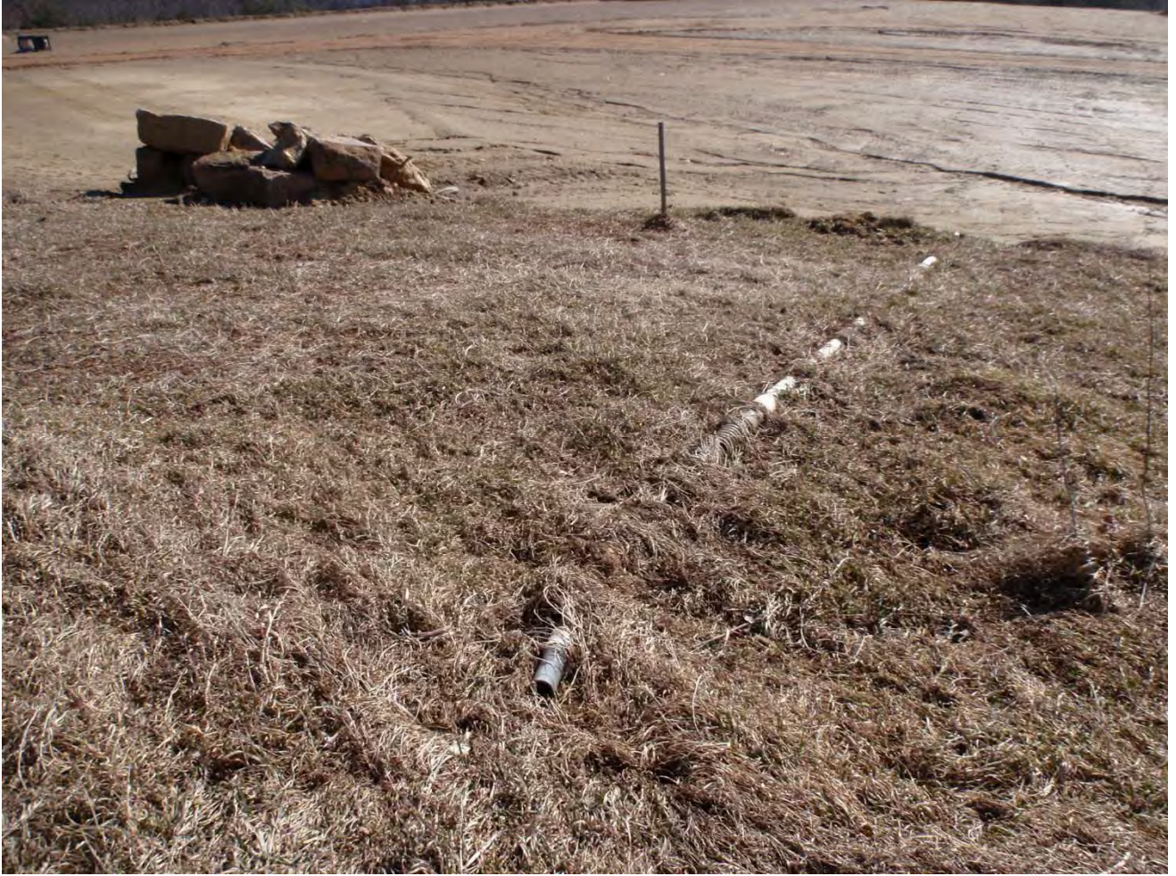
Abandoned Header near Former EW-19
