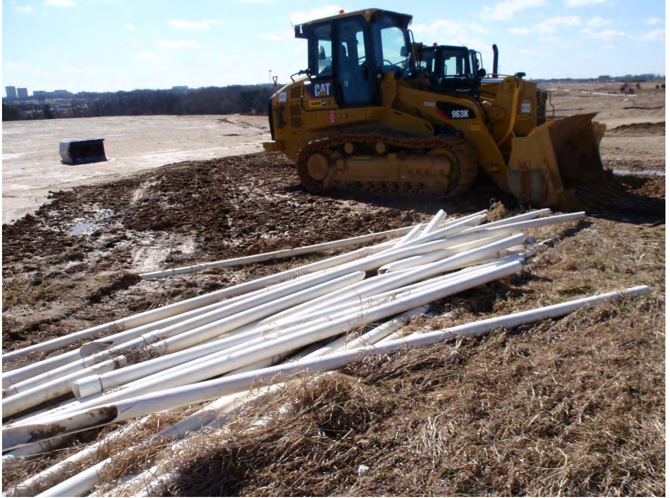
Abandoned Header near Former EW-20
