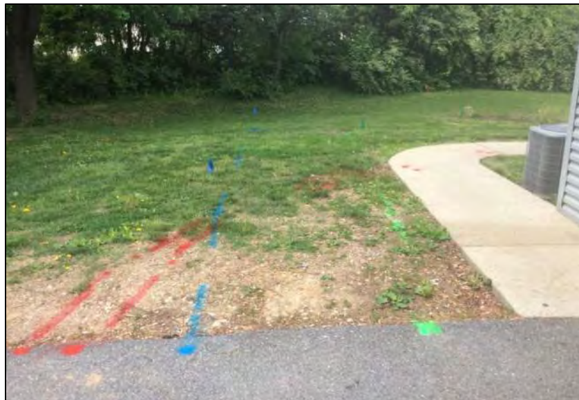
Figure 2: Example of field mark out, picture depicts a section in Area 1 (near homeless shelter) where two (2) electric lines cross over a water and storm drainage lines.
