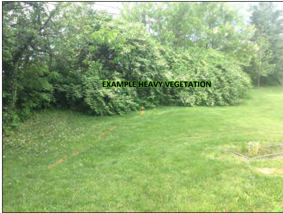
Figure 4: Section of Area 1 on Sheet 2 where the communication, electric and storm drainage intersect the area of heavy vegetation called out on the utility mapping.
