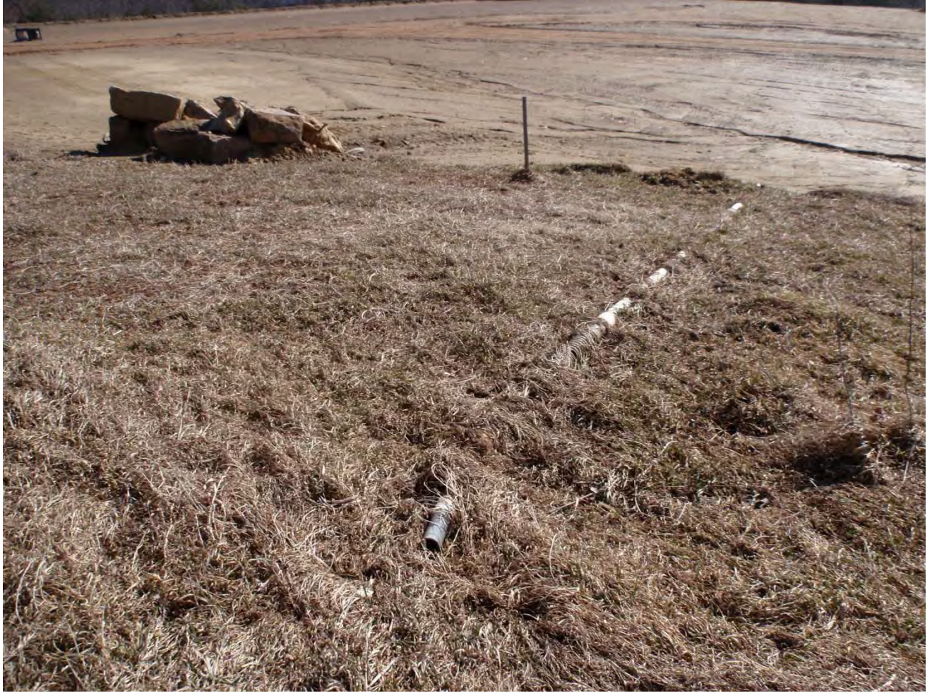
Abandoned Header near Former EW-19
