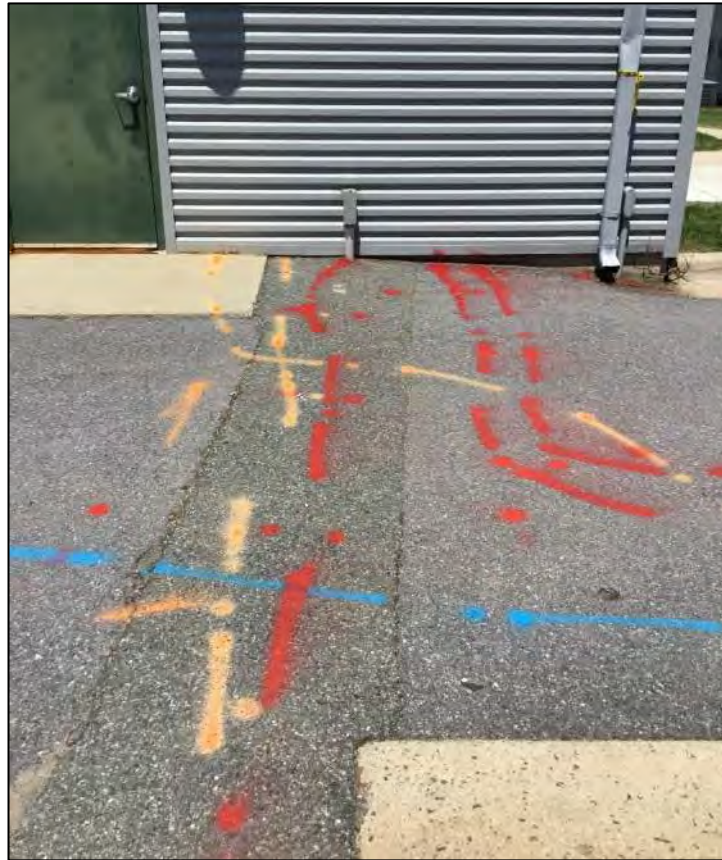
Figure 3: Example of field mark out, picture depicts a congested section in Area 1 (near homeless shelter) where three (3) electric, two (2) communication and one (1) water line converge.
