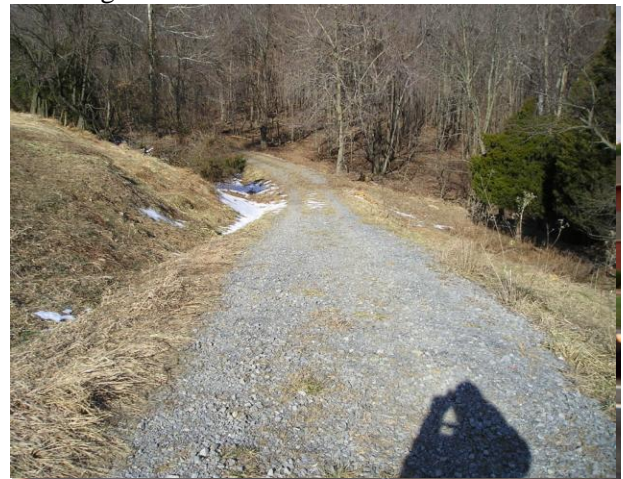
6. View of access road to proposed location for MW-2A/MW-2B facing north.
